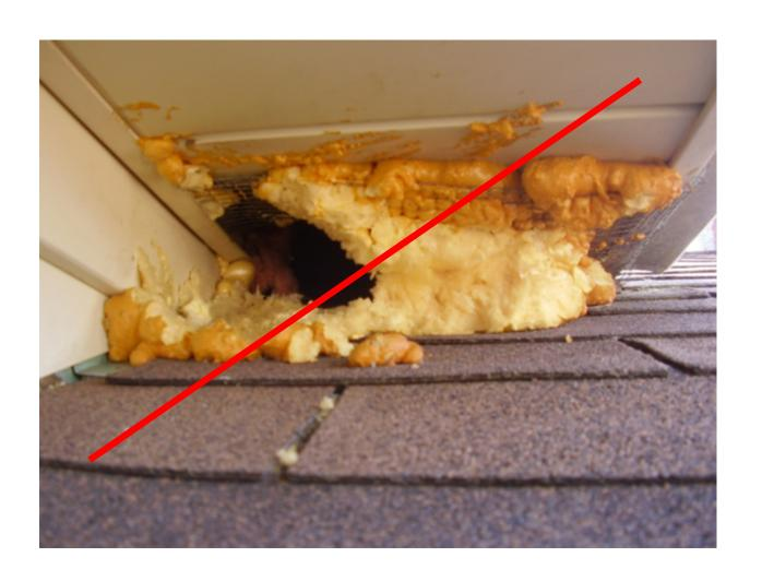
Use it with metal mesh or flashing and seal with concrete
