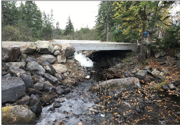
New bridge to enhance fish passage at Cold Stream Forest Unit, BPL Western Region
