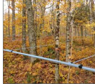
A portion of maple sugar collection system installed on license area
