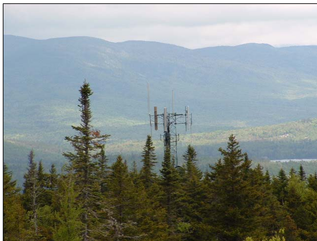
View of the Communications Tower on Bald Mountain from the hiking trail near summit
