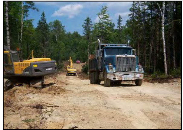
2011 Management Road Construction at Nahmakanta
