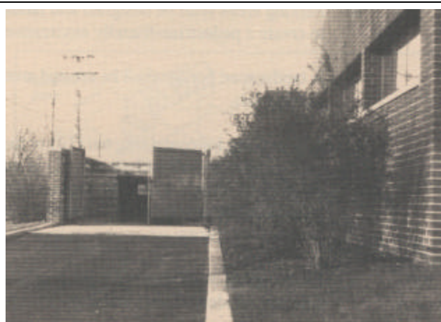
A good example of a dumpster placed on an impervious surface and screened from view with a high brick wall and gates.
