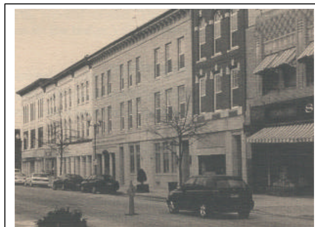
The windows in the central, new building match those of the buildings on either side.
