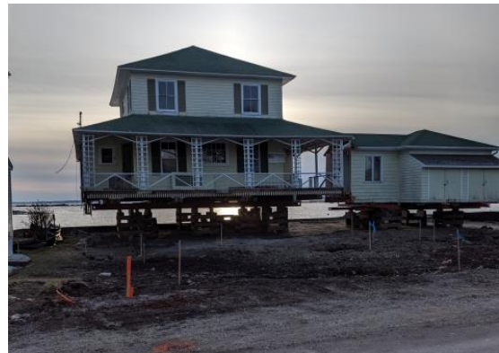
A Beach Avenue home being lifted onto a higher foundation in 2020 Photo credit: Janice Vance
