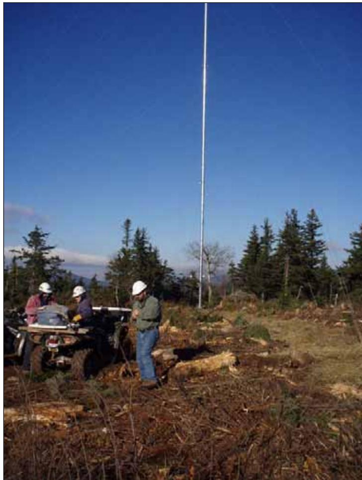
Figure B-3b: A tubular structure with guys and mulched guy corridor
