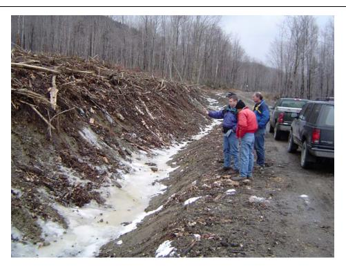
Photo 7: Recently built existing road cut across moderately well drained soil exhibiting seepage on top of soil underlying glacial till. Erosion and sediment control not yet in place. Photographed by A.F. 11/12/2003.
