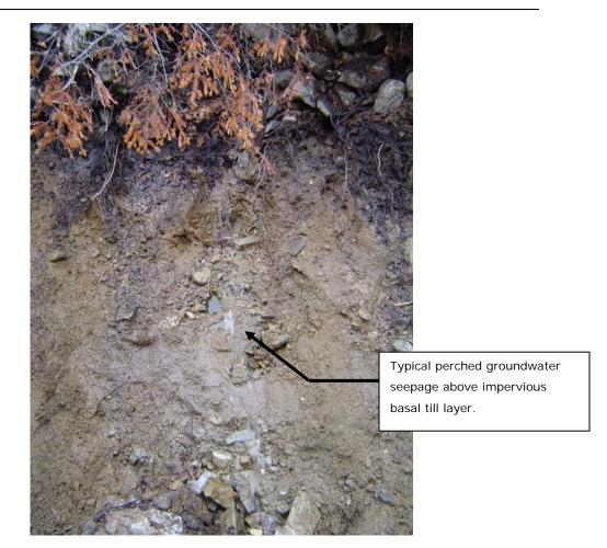
Photo 6: Ground water seepage. Photographed by A.F. 11/12/2003.
