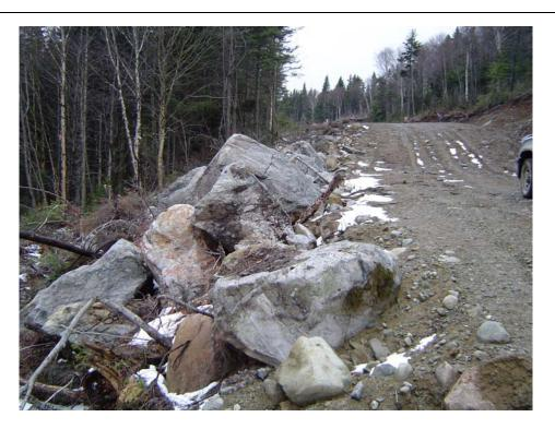
Photo 9: Large boulders utilized on downslope side of fill extension for fill retainment and rip rap armament. Photograph by Albert Frick, 11/12/2003.
