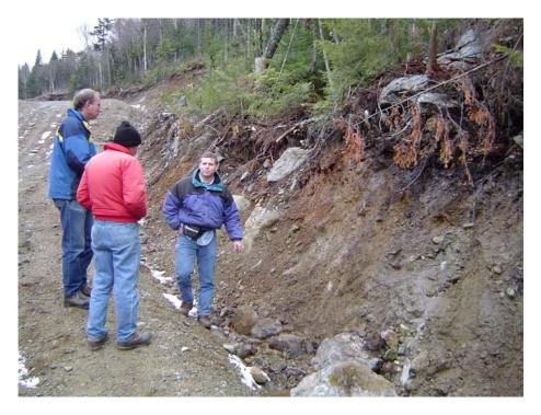
Photo 8: Boulders and cobbles encountered on surface shall be utilized to downslope fill extensions. Photograph by Albert Frick, 11/12/2003.
