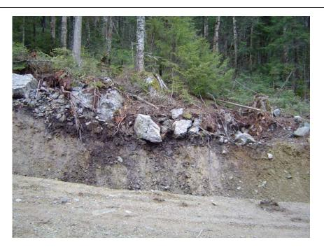
Photo 2: Existing high elevation road cut at Seven Ponds TWP at 2,600'+/-. Photo illustrates typical strong surface horizon over glacial basal till substratum. Location not in project area, however, used as available example of deep road cut in high elevation mountainous area, exhibiting typical very stony soil surface over firm basal till. Photographer A.F. 11/12/2003.
