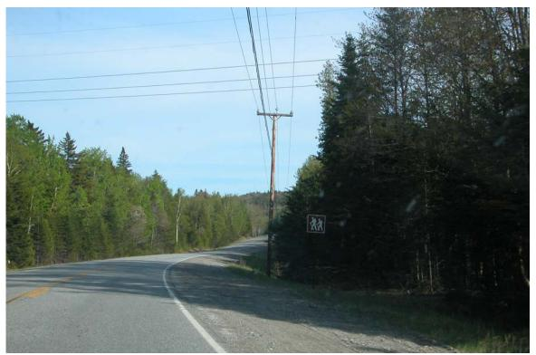
6-P78: Route 27 looking southeast at the Appalachian Trail crossing. Existing overhead 34.5 kV distribution lines (running parallel to the road) extend into Stratton. Existing overhead 115 kV Boralex transmission lines (running perpendicular to the road) tie into the Bigelow Substation located behind the trees on the left.
