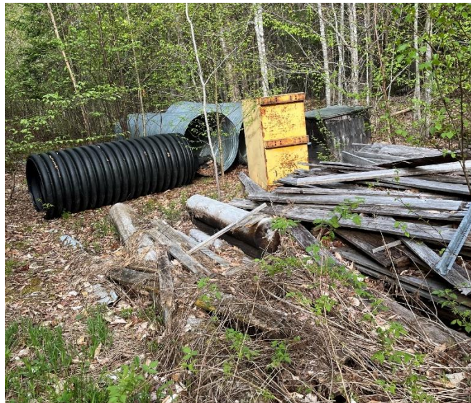
Figure 4: Remaining Materials on Site
