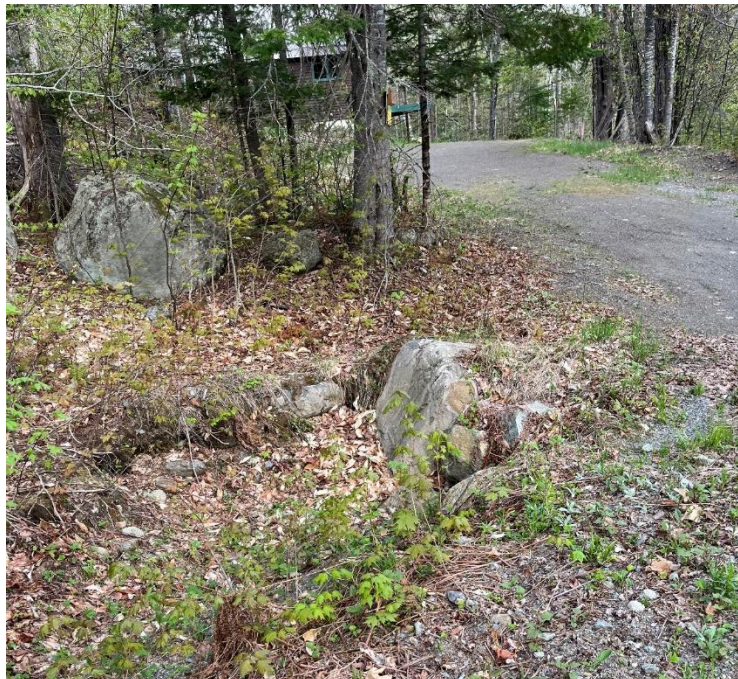
Figure 6: Entrance to Existing Building
