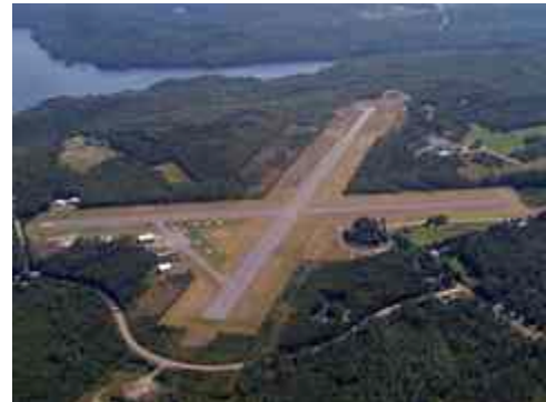
Greenville Municipal Airport
