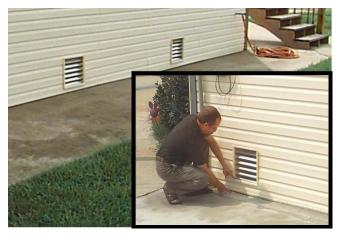
A code inspector measures height of flood vents which allow floodwater to flow underneath a building.
