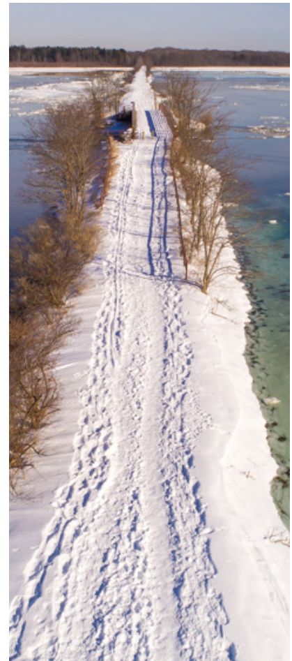
Photo Credit: Dave Cleveland under contract to Town of Scarborough
