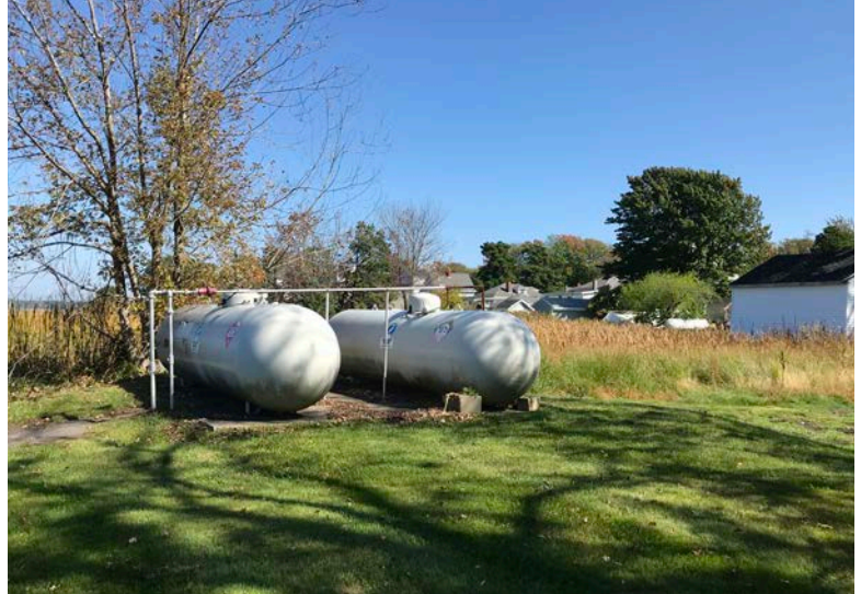
Left: Highly volatile gas tankers being stored in high hazard area adjacent to the marsh. Right: Propane tanks installed within feet of the marsh can become a deadly threat to people and property during flood events.
