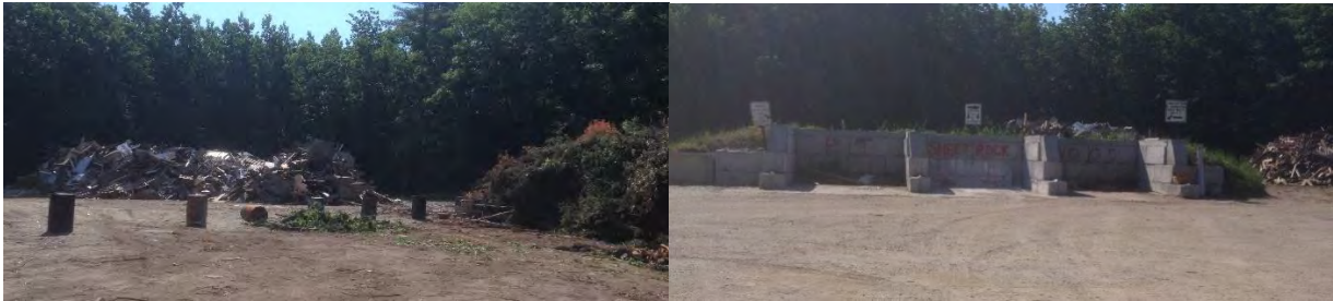
Demolition and Waste Wood Disposal Area and Revetment
