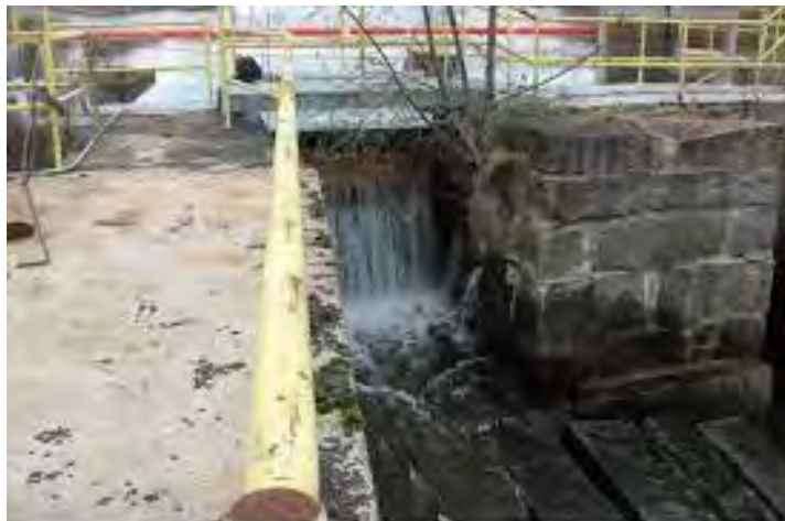
Thompson Lake Dam
