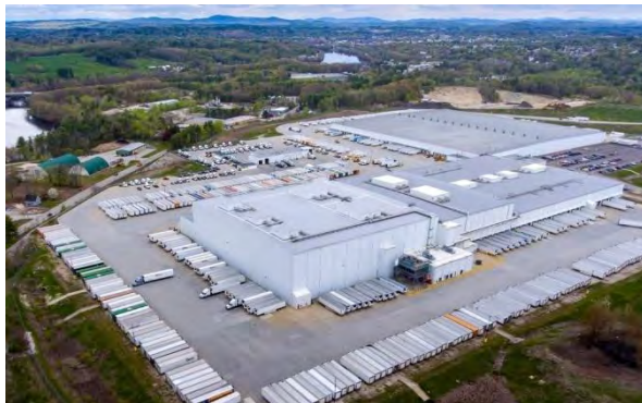
Wal-Mart Distribution Center, Lewiston
