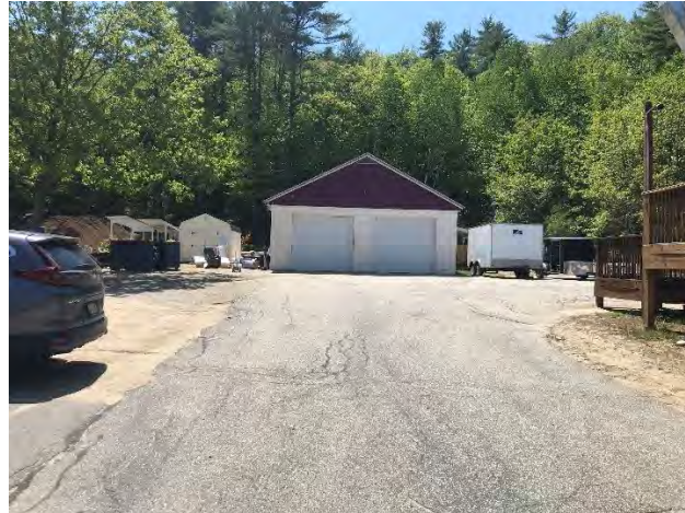
Old Fire Station/Recreation
