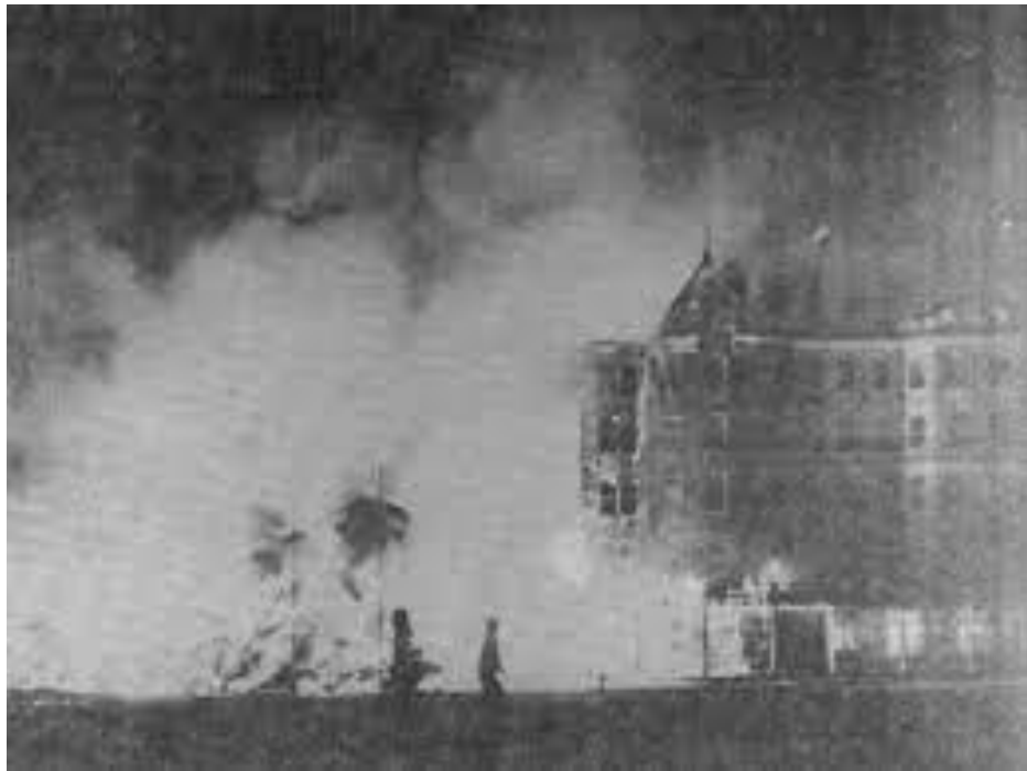
Poland Spring House Fire
