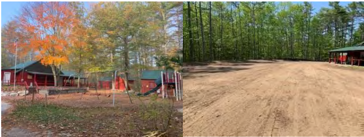
Camp Connor Main Building Front and Rear View (the berm has just been removed)
