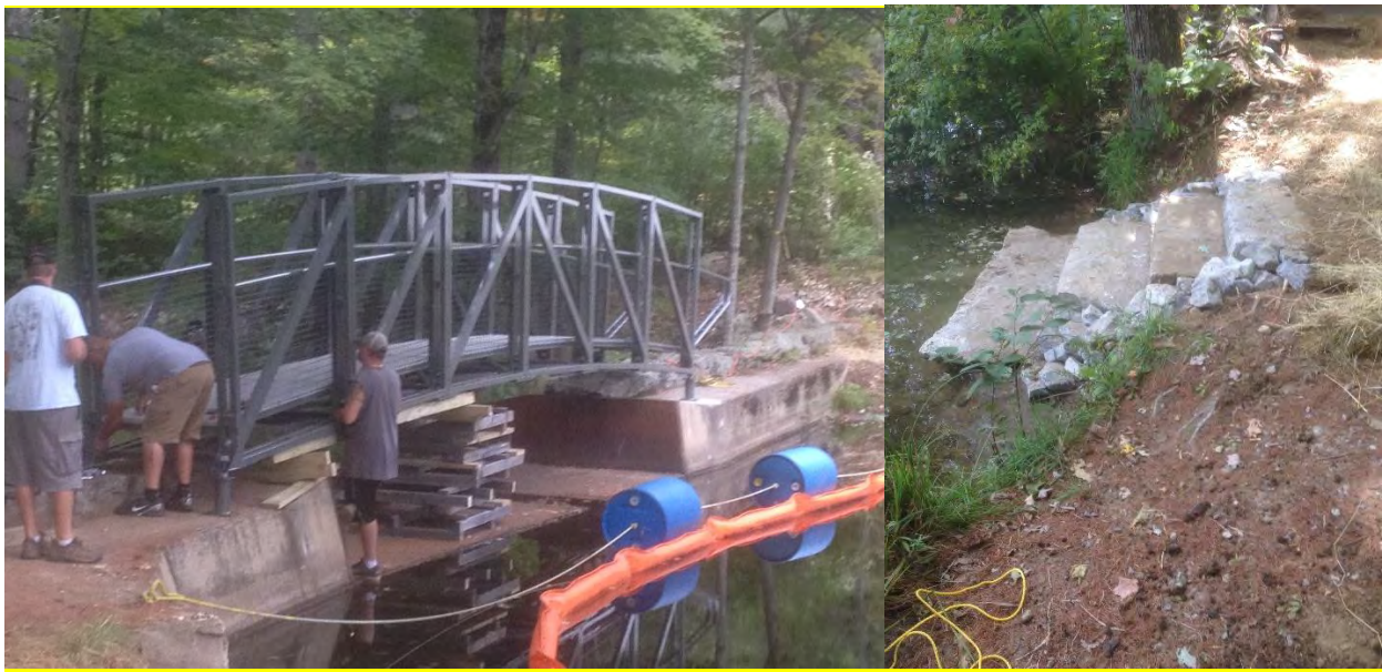
Waterhouse Brook Bridge Installation and Canoe/Kayak Landing
