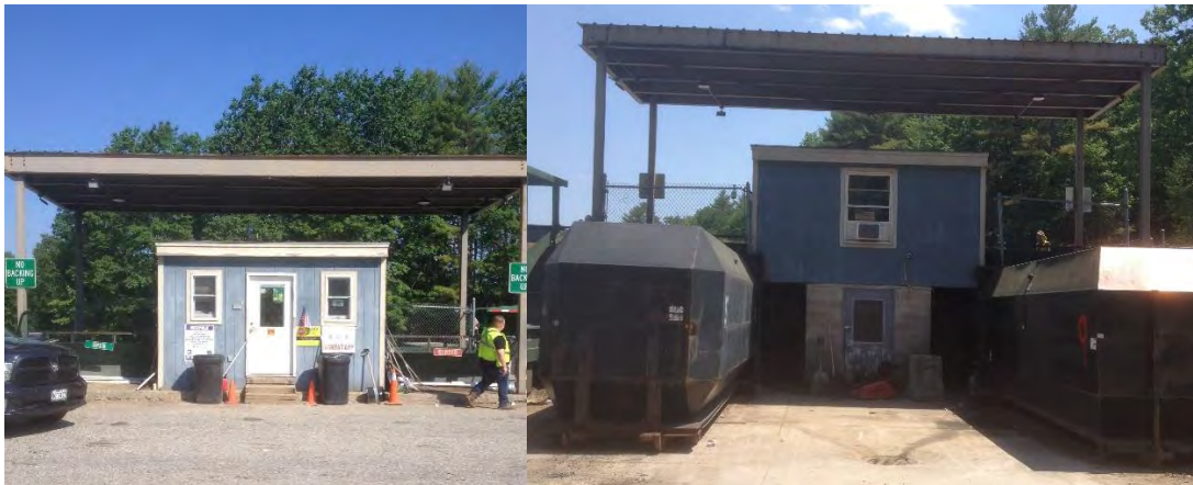
Transfer Station Main Office and Trash Disposal Area – Front and Rear View
