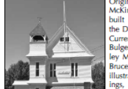
[14] Seamark Building Church Street
