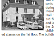
[13] Masonic Hall Church Street
