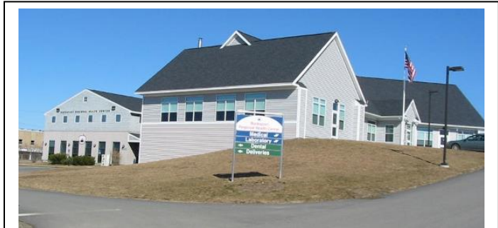
Bucksport Regional Health Center on Broadway has offices for primary medical care & dental services and lab facilities. A major addition was added in 2013.
