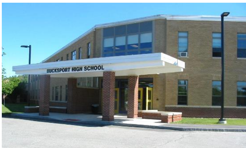
Bucksport High School got a very much needed face lift in 2014 with funding through the regional school unit. The insulated and air tight brick replaced the leaky 1960's glass block façade at a cost of more than two million dollars.
