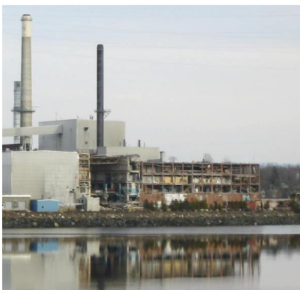
Paper mill demolition Phase I, Feb. 2016
