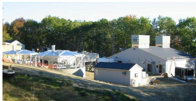
Wastewater Treatment Facility under construction in 2016
