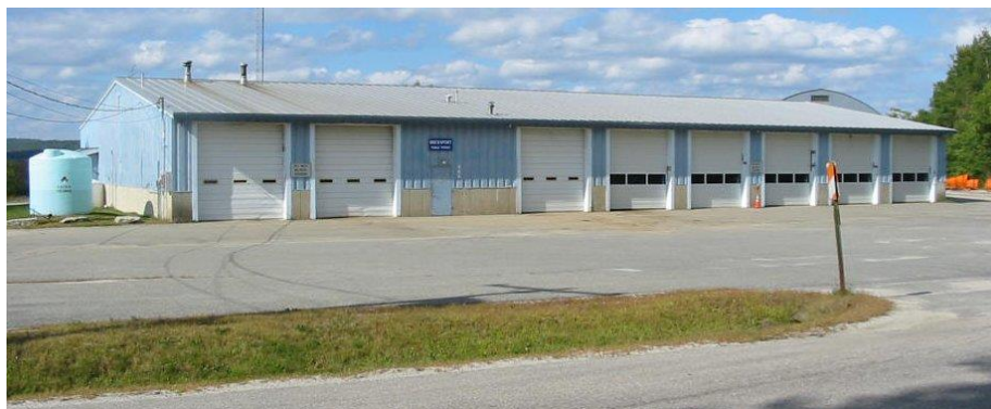
The Highway Maintenance Garage at 360 Central Street
