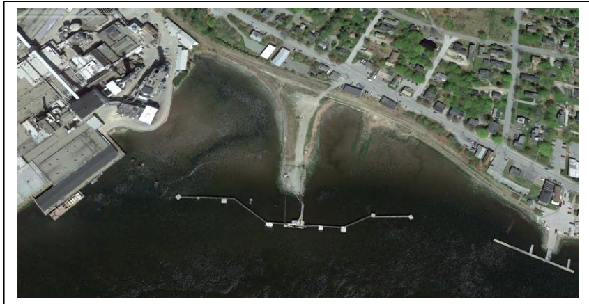
The mill site, the Webber Dock (formerly called Sprague South) and the extended town pier form the western end of the town harbor.
