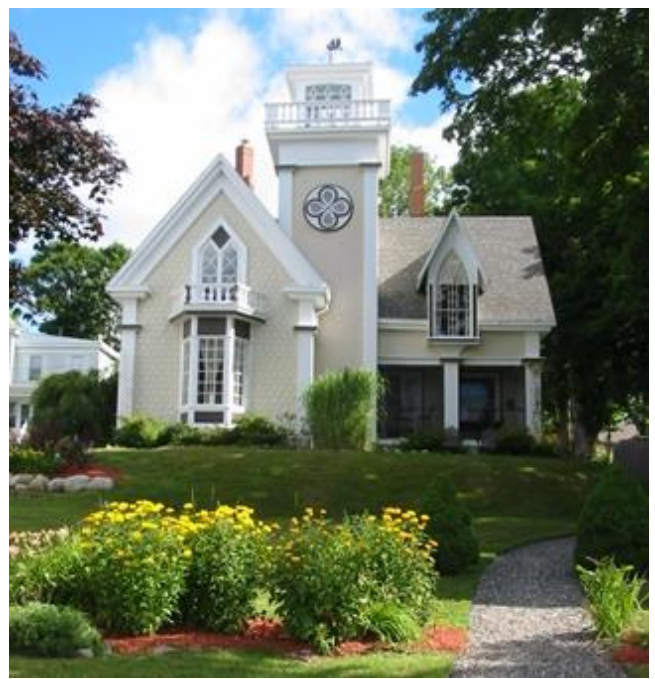
Emery House - Linwood Cottage at 101 Main St, with its restored tower, is listed on the National Register.
