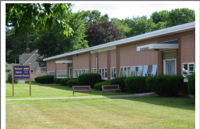
The Parks and Recreation offices, conference room, gym and exercise facilities are in the Jewett School on Bridge St.
