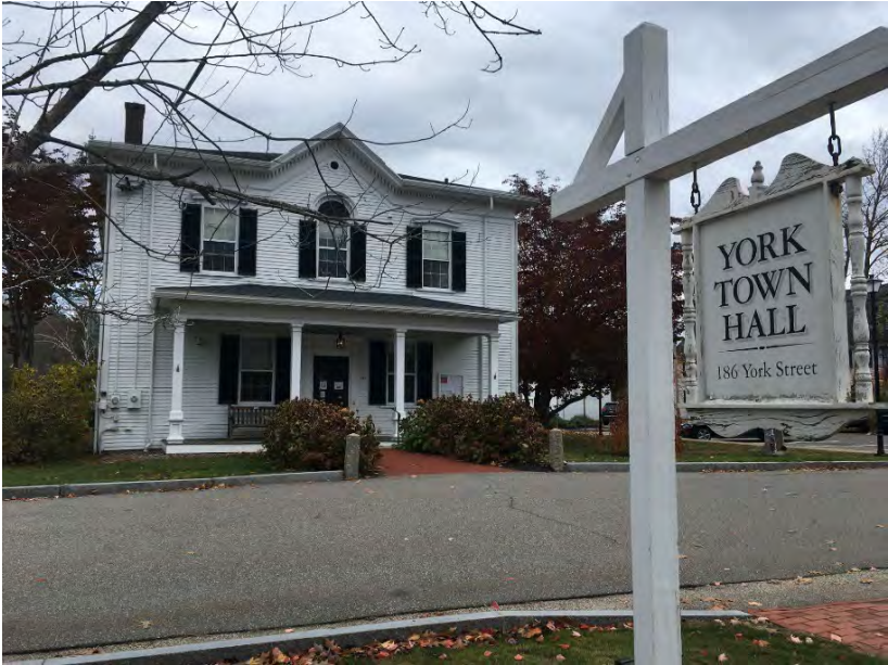
York Town Hall, existing facility 2022.
