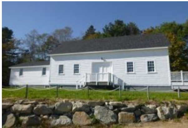
Relocated museum in place and secured
