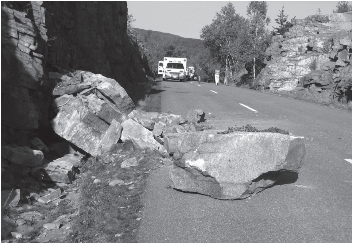
▲ Figure 3. Rockslide onto the park loop road in Acadia National Park due to the MLg 4.2 earthquake on 3 October 2006.
