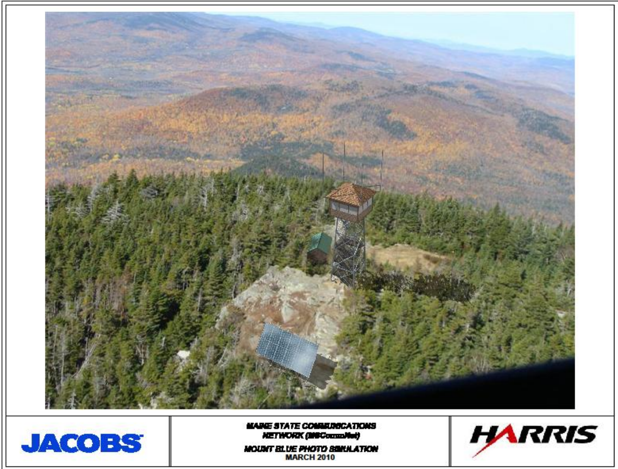
Figure 4: Artist conception of new Mt Blue public safety radio communications tower (aerial)
