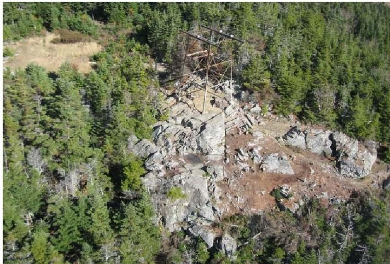
Existing (Abandoned) Fire Lookout Tower
