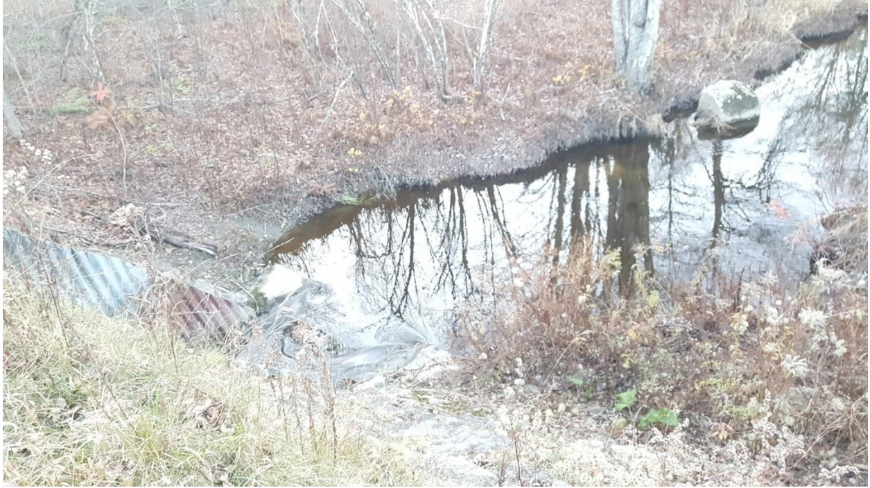
Figure 10. Upstream end of existing culvert, note drop into culvert from upstream pool.
