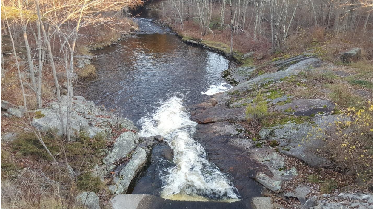
Figure 6. Looking downstream. Note drop at lip of culvert concrete pad.
