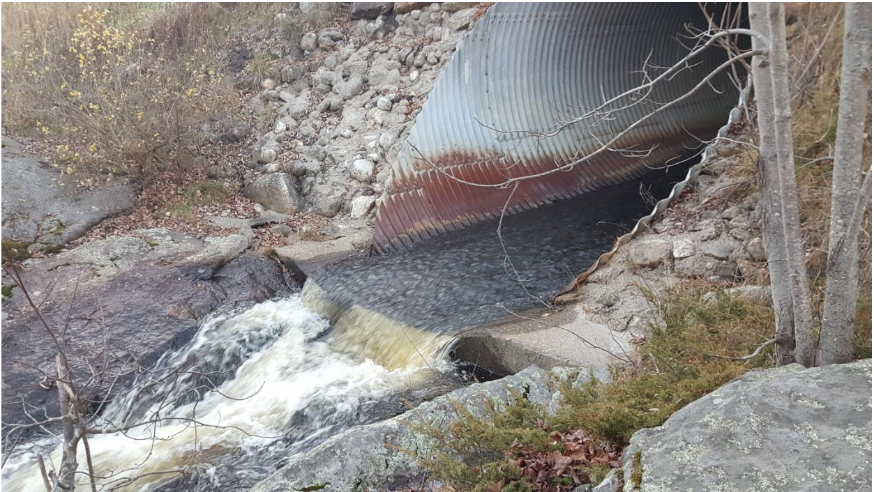
Figure 7. Drop at downstream end of culvert.
