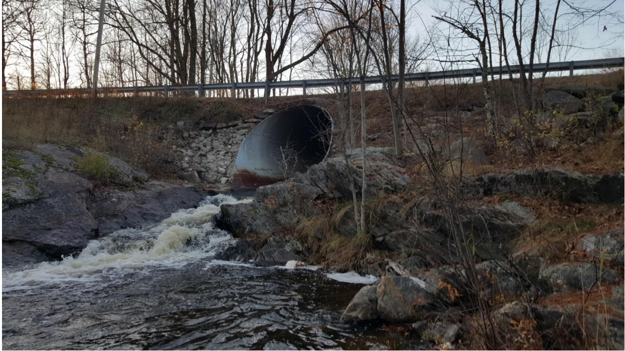
Figure 4. Downstream Face. note sharp drop below culvert into pool.
