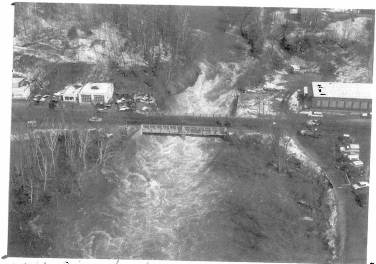
Webb River bridge over Webb River - Dixfield - Mexico May, Sh 87-2 4-2-97
