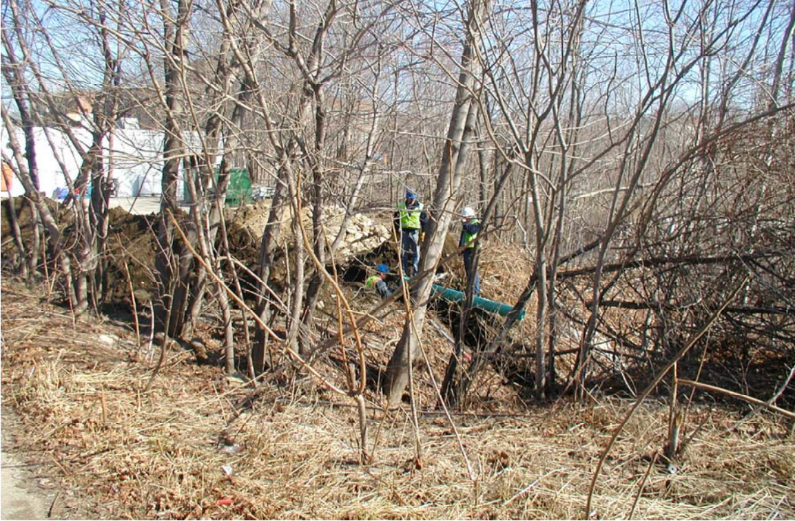
Route 1 - Brown Street Drainage 005
