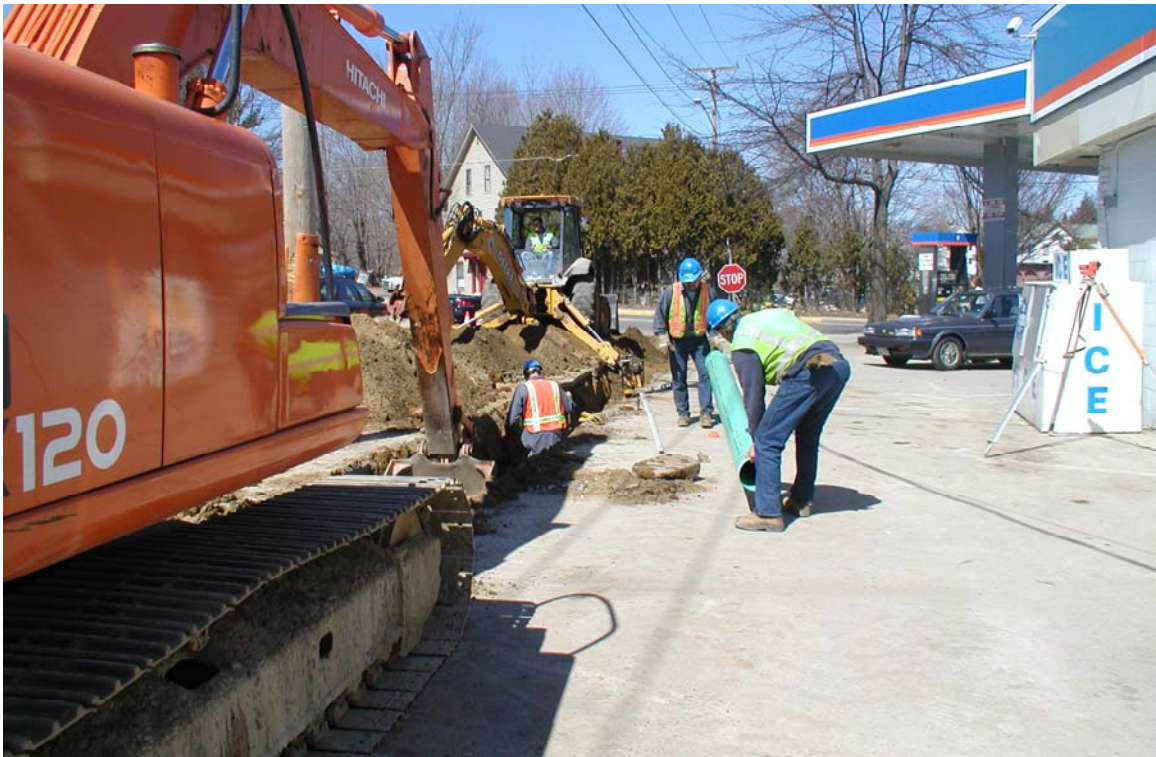
Route 1 - Brown Street Drainage 008
