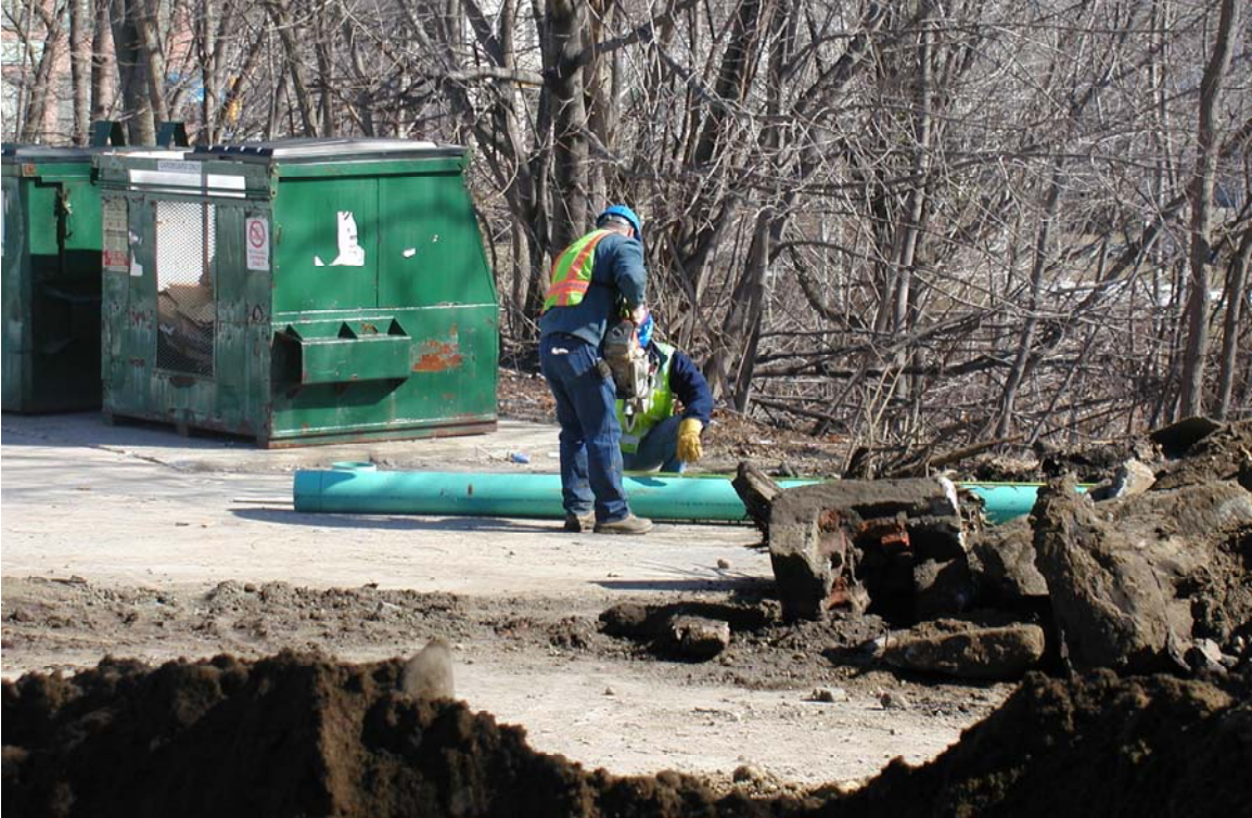
Route 1 - Brown Street Drainage 001
