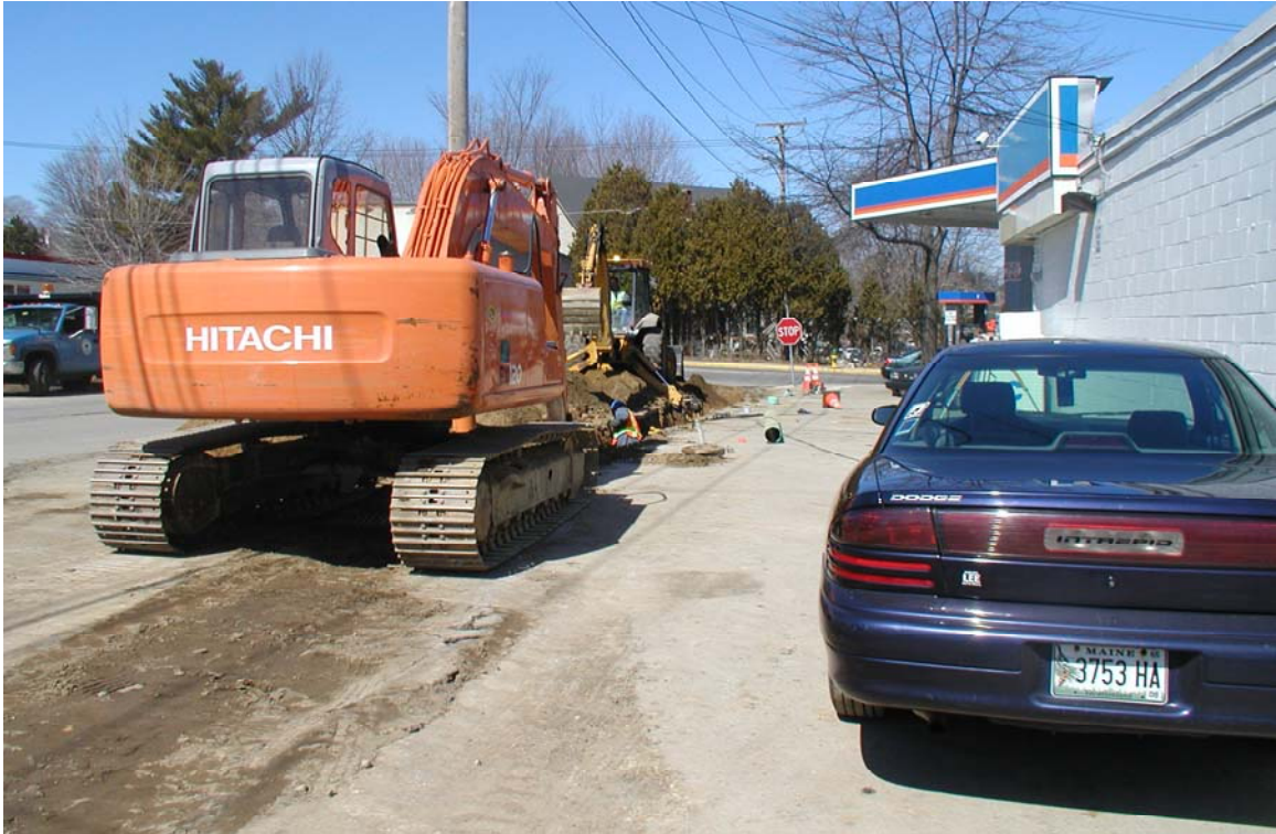
Route 1 - Brown Street Drainage 007
