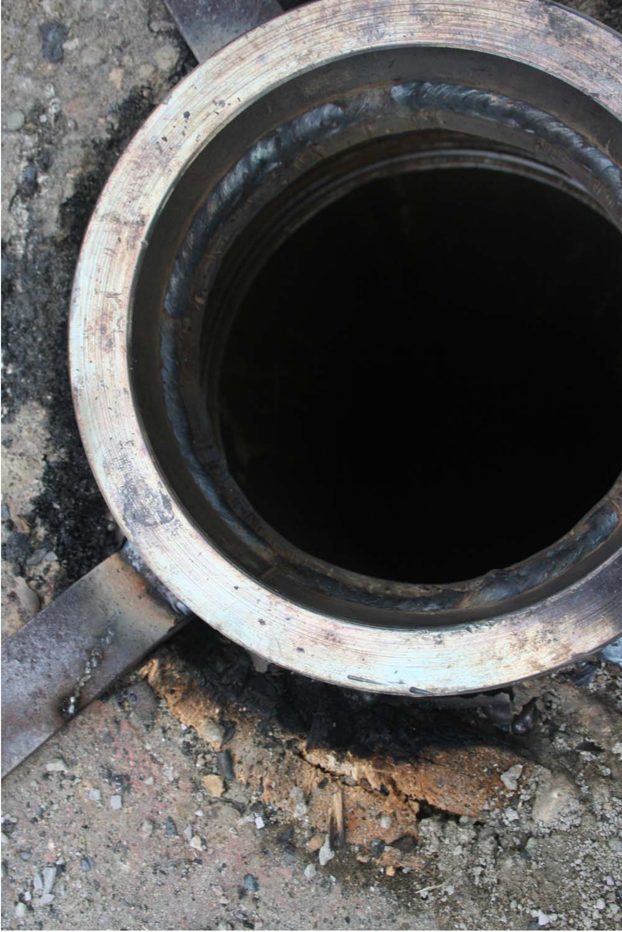
Route One Sinkhole Repair – Kennebunk 11-7-2006
