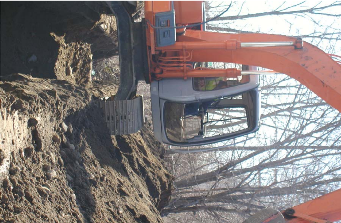
Route 1 - Brown Street Drainage 002
