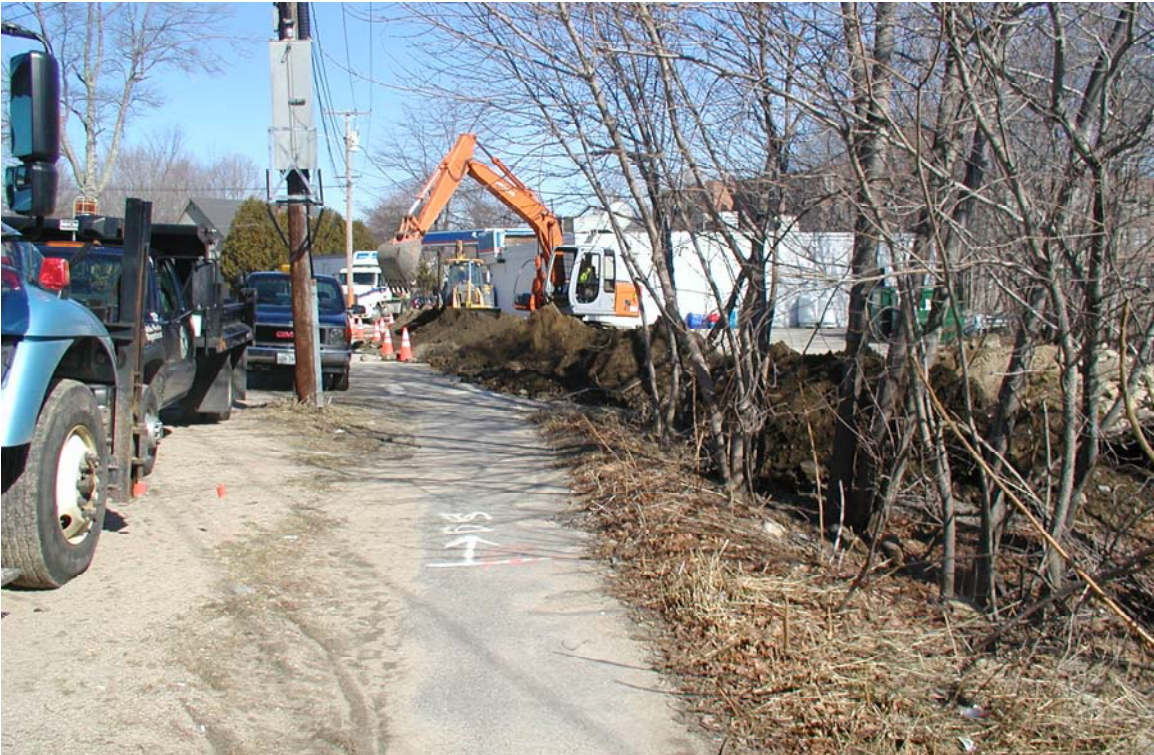
Route 1 - Brown Street Drainage 006
