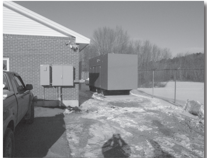
New Generator at Berwick Water Department
