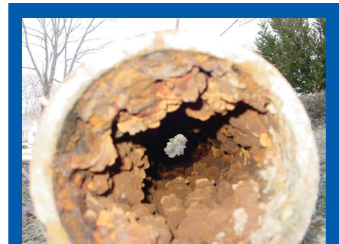
Minerals can build up in old water mains, leading to pressure and bacteriological problems. Pipe can be replaced, or it can be rehabilitated using a "pig" to scour the inside of the pipe and remove the deposits
