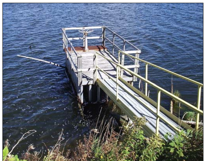
The outlet structure on the south end of Christina Reservoir allows constant overflow to Prestile Stream.
