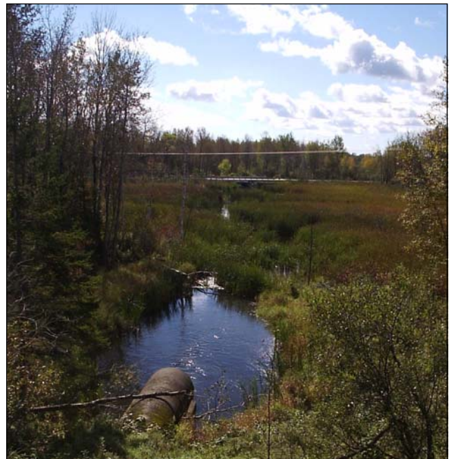
Prestile Stream (looking downstream) flows out of Christina Reservoir through a culvert.
