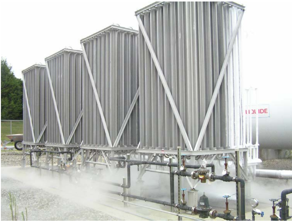
Figure 2: Oxygen Supply Facility Ambient Air Vaporizers
