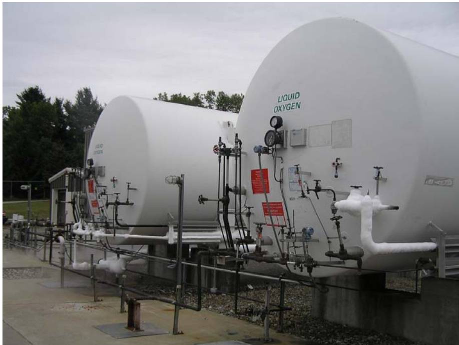
Figure 1: Oxygen Supply Facility Storage Tanks
