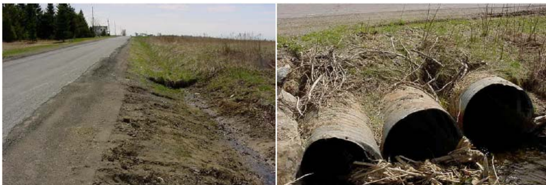
Examples of common roadway problems in the Trafton Lake Watershed. Roadside erosion (right) which transports sediment to streams that feed Trafton Lake can be reduced by regular maintenance (grading) of road shoulders and removal of winter sand/salt. Cleaning out clogged culverts (right) and armoring the inlets with rip rap can reduce flow problems and erosion at culvert inlets/outlets (Easler 2002). Proper design and maintenance of roadside ditches can help reduce erosion and sedimentation.
