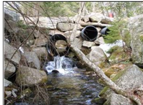
Before: Failing culverts contribute erosion issues into a stream that empties into Branch Lake.
