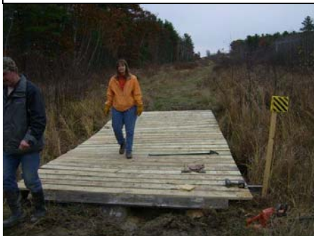
After: Volunteers repaired bridge and stabilized approaches with crushed stone. Large boulders and signs installed to discourage future stream access.
