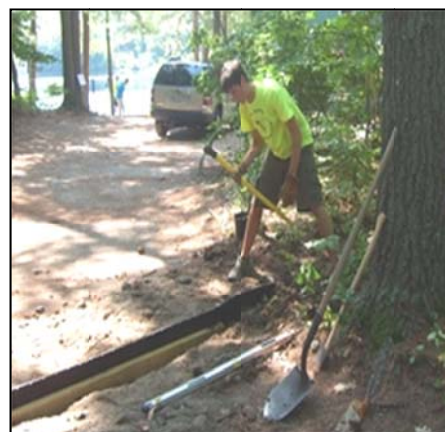
YCC crew members help protect water quality one conservation practice at a time.
