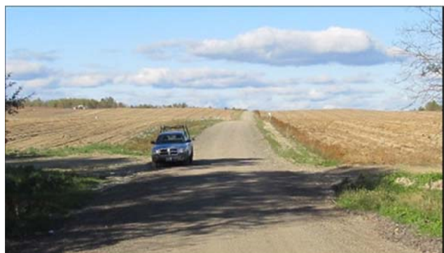
Town road with a grass-stabilized ditch
