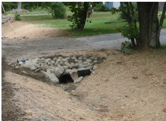
An example of a BMP installed on Woodland Ave to prevent erosion and sedimentation.
