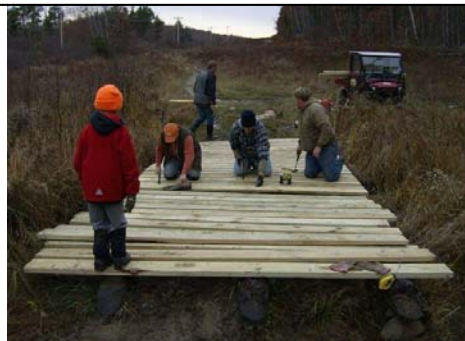
After: Volunteers repaired bridge and stabilized approaches with crushed stone. Large boulders and signs installed to discourage future stream access.
