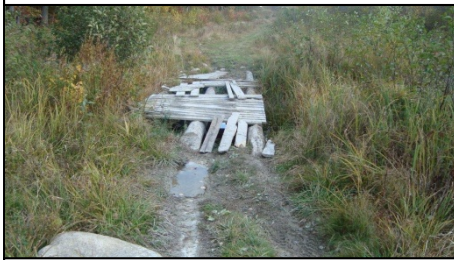
After: Volunteers repaired bridge and stabilized approaches with crushed stone. Large boulders and signs installed to discourage future stream access.
