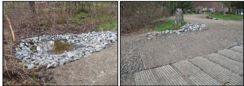
After – culvert outlet armored, road runoff redirected through super elevation, and stabilization of ramp with cement planks
