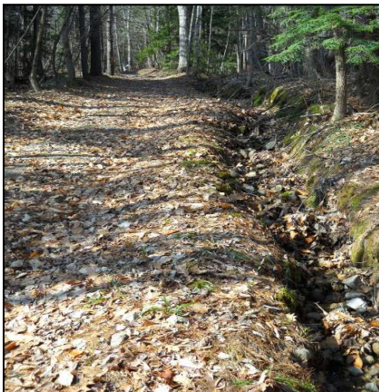
Before – This unpaved road was identified as a high impact problem. Erosion from the road surface and ditch washed directly into Thompson Lake.
