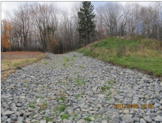
Rock-lined waterway discharging into a small pool with a level lip spreader that discharges into a riparian buffer.
