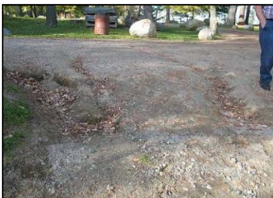
Before – Boat ramp erosion
