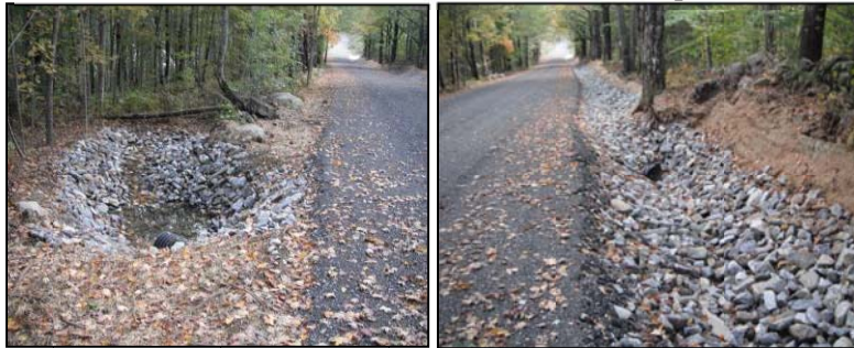
Work in this roadway included ditch installation, riprapping, and installation of turnouts and sediment pools
