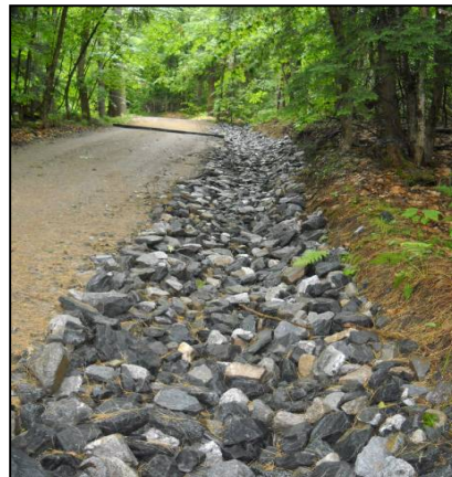
After –The road was crowned and a rubber razor was installed to shed water to the ditch. The ditch was reshaped and stabilized with angular rocks.
