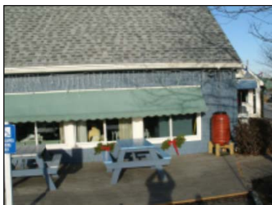
Rain barrel installed at Bob's Clam Hut
