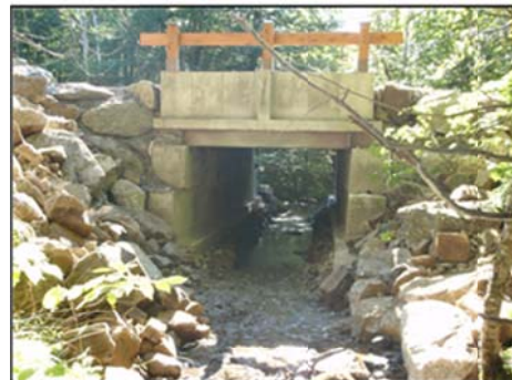
After: A new bridge reduces erosion issues and sediment getting to the lake.
