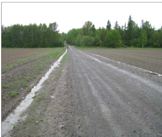
Town road lacking a stabilized ditch
