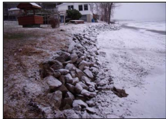
Shoreline stabilization project
