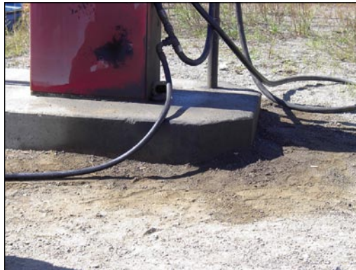
Spills to gravel.
