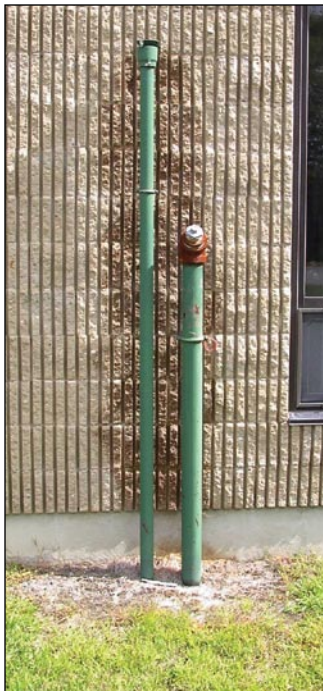
Overfill spill into soil.
