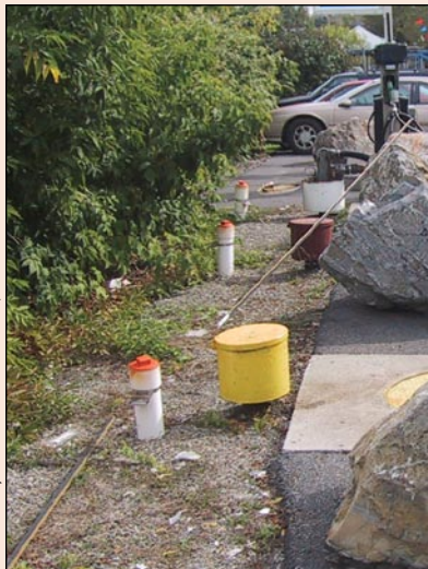
Above-grade spill buckets.
