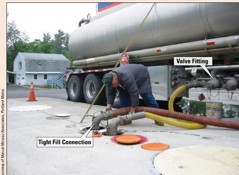
When your UST is full of fuel and the driver's hose is full of fuel that won't fit in the UST, the driver has an overfill situation.
