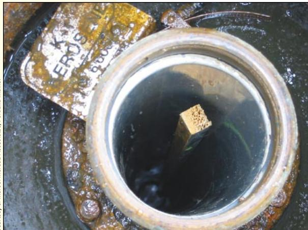
**Gauge sticks in fill pipes prevent drop-tube shutoff valves from operating. They are illegal and can result in overfills.**
