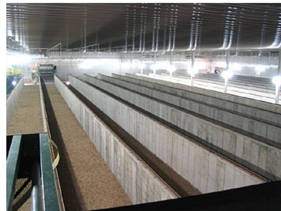
Agitated bins, Delaware Co., NY
