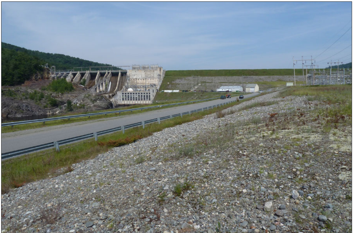
Photo 14. Wyman Dam just below the lake
