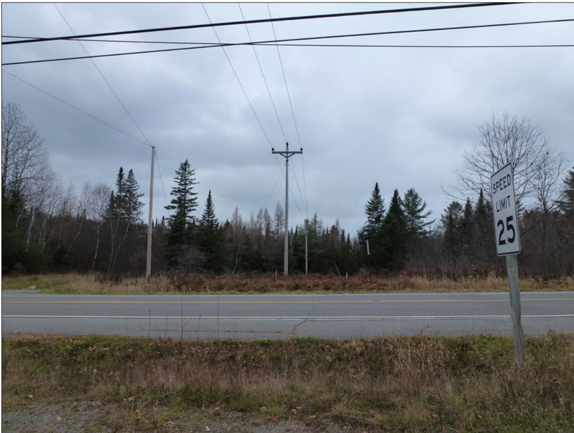
Photo 35. Existing transmission line that feeds into the Guilford substation
