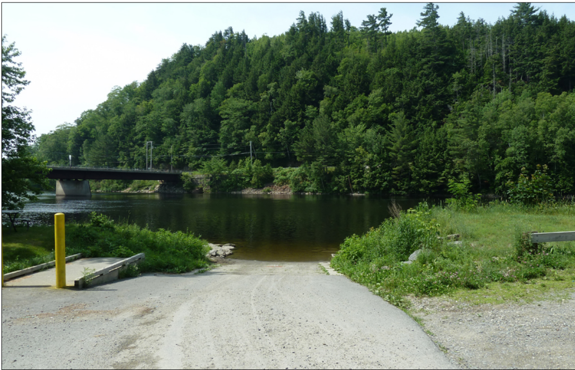
Photo 11. Boat launch located just north and east of the bridge
