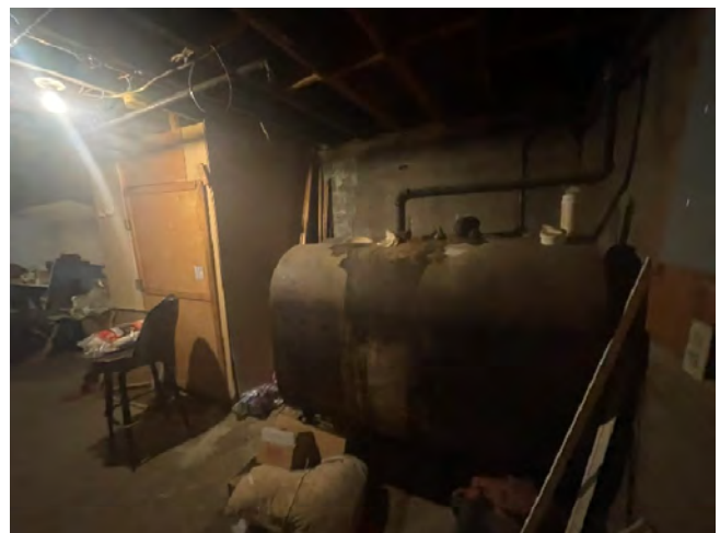
Description: Photo Studio Basement, AST location.
