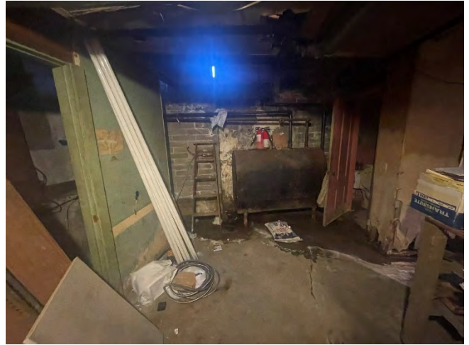
Description: Pawn Shop Basement, Sample AS-2 location
