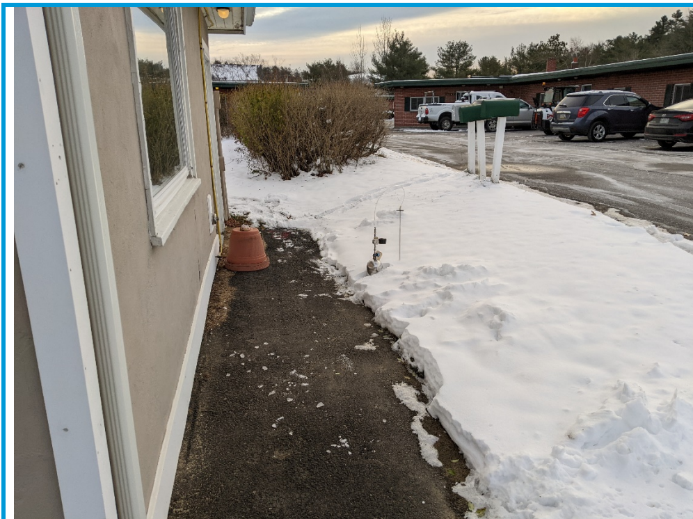
Photo No. 2 Site Location: 211 US Route 1 Falmouth, Maine Photo Date: December 21 2021 Description: SV-102 to the south of the Lazy Bones building. Photo By: JKC
