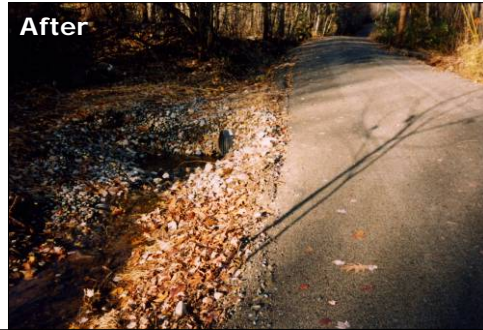
Loon Nest Estates Road – Prior to construction, runoff was trapped on road, which led to erosion of the road surface. Project resurfaced and shaped road and installed ditches.
