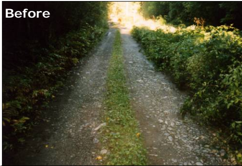
Loon Nest Estates Road – Prior to construction, runoff was trapped on road, which led to erosion of the road surface. Project resurfaced and shaped road and installed ditches.
