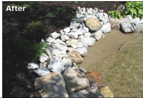
BRCA Conservation Corps stabilized eroding shoreline with riprap and buffer vegetation
