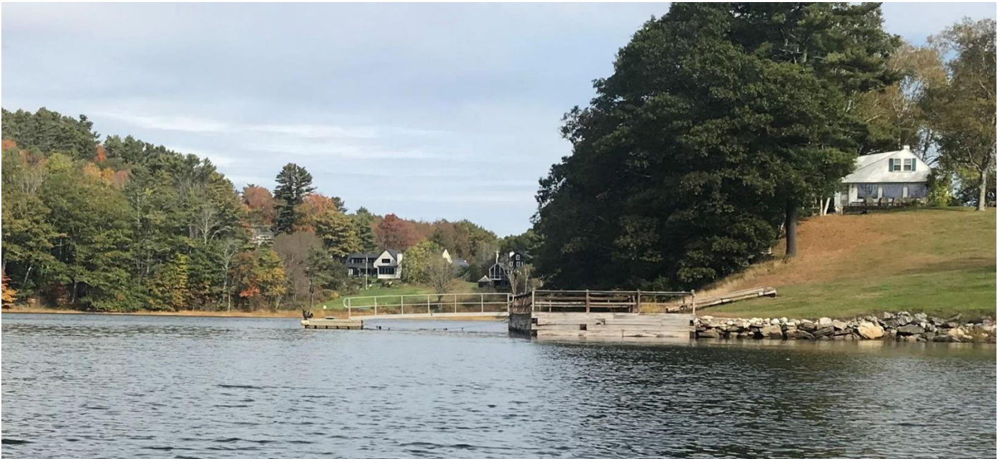
Photo 85: Large permanent 26x84 wharf (old mill), 3x30 ramp & 12x20 float - Davis - In 1924 the dam was dynamited to facilitate access by boats to the upper river. 22' wooden power boat normally here.
