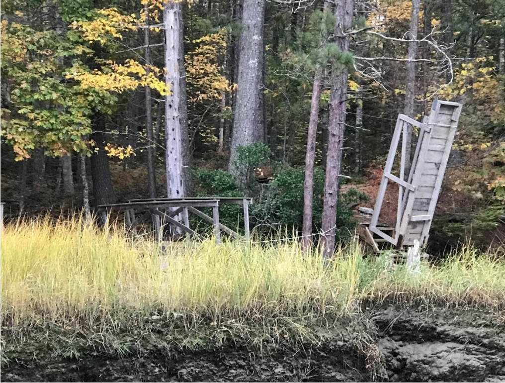
Photo 17: Lifted wooden dock/pier/floats with permanent concrete piers below HAT - (formerly Bill Mook) - Now Leah Sprague - commenter
