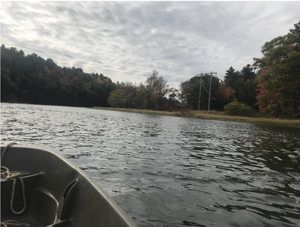
Photo 41: CMP powerline crossing
