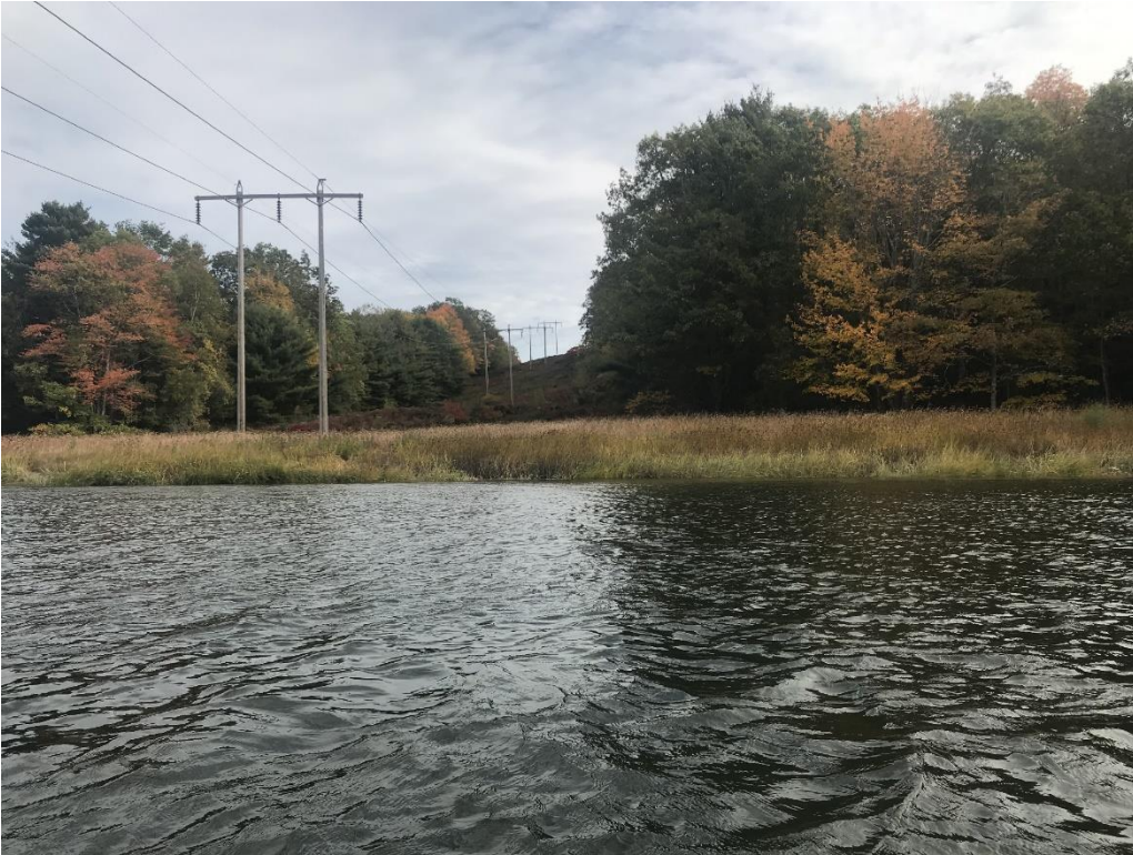
Photo 43: CMP powerline crossing
