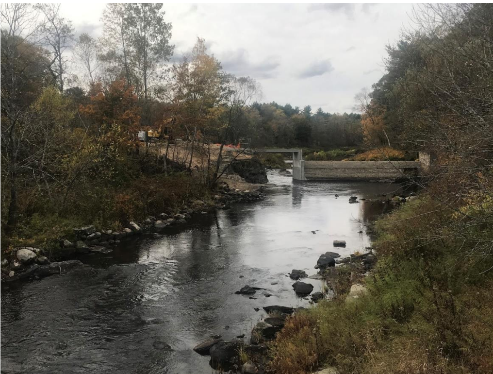
Photo 4: Head Tide Dam, views up and down river, and parking, and stairs. NOT YET COMPLETE
