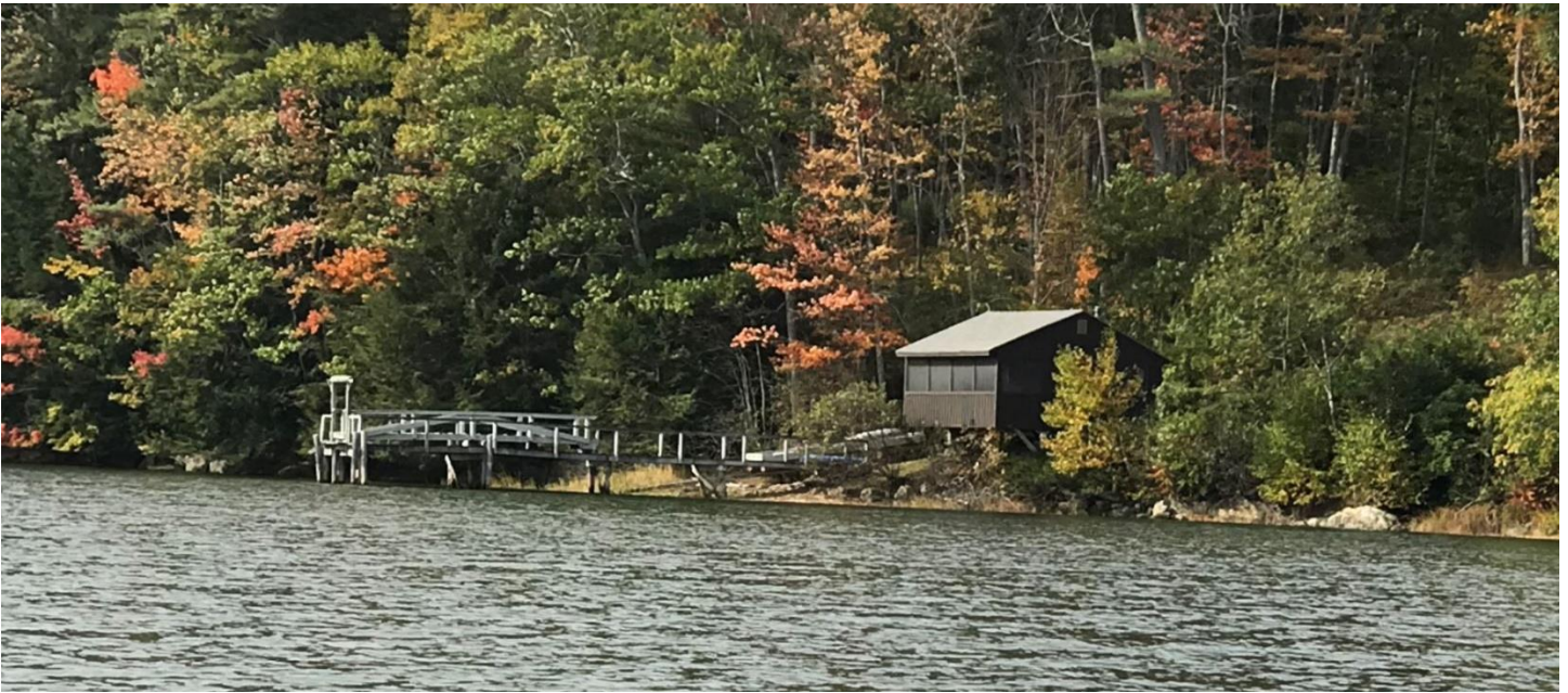
Photo 75: Permanent pier 5x60, 4x32 ramp, 10'x20' float - R. Colby
