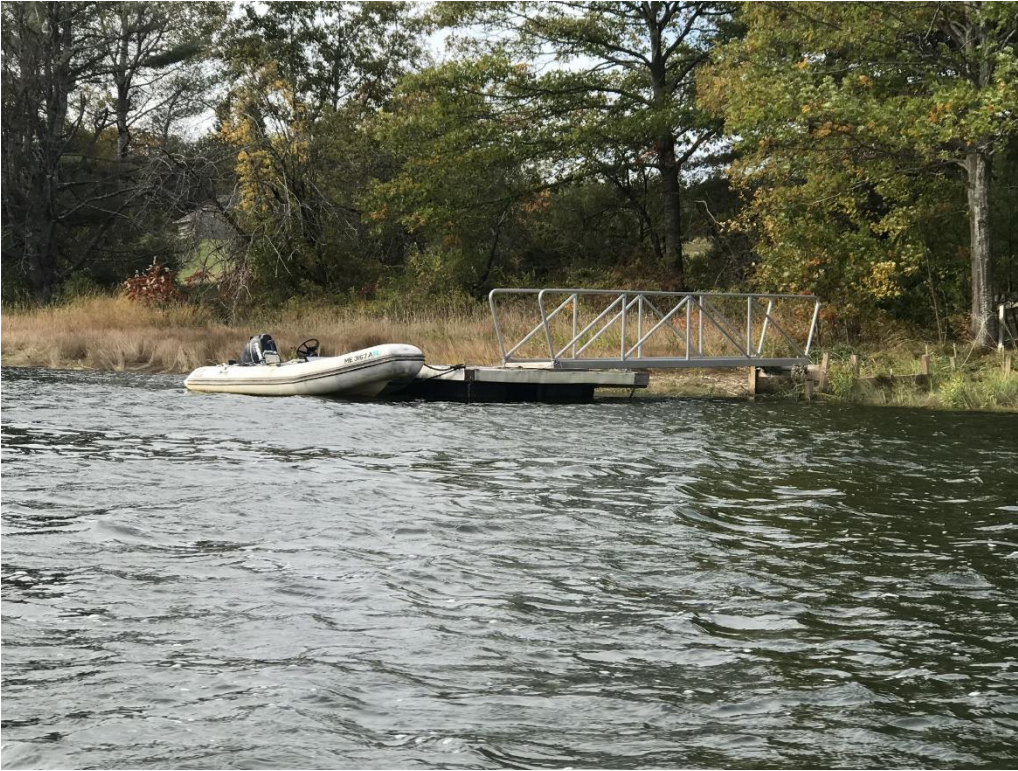
Photo 71: Whittemore - Dock w/ upland piles, ramp, float and ~16' zodiac center console (left hand) - Whittemore
