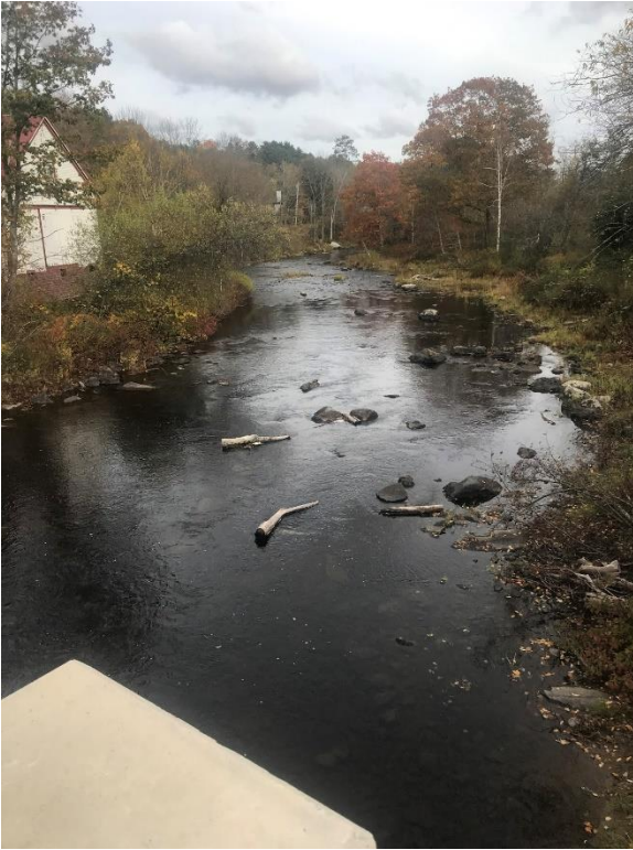
Photo 5: Head Tide Dam, views up and down river, and parking, and stairs. NOT YET COMPLETE
