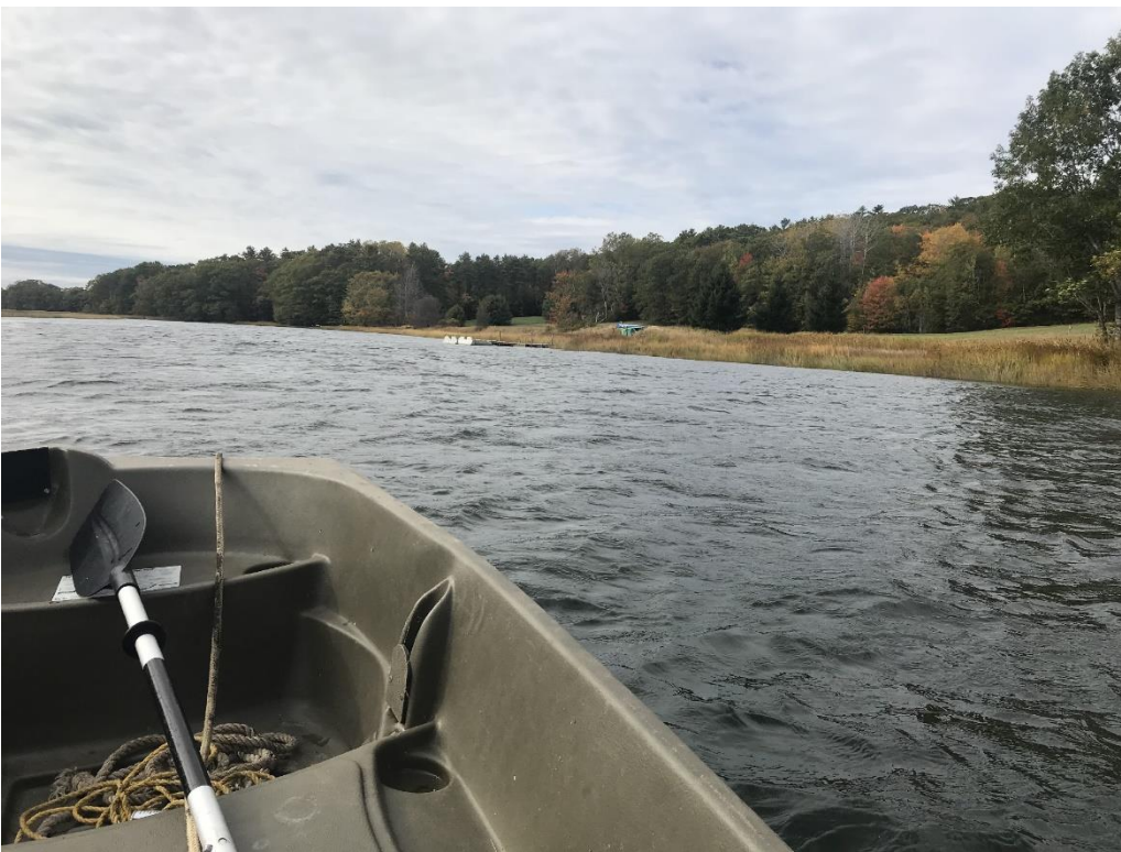
Photo 20: Hana - dock 60' gangway w/ piles, 10x10 float, attached kayak launching float ~4x10
