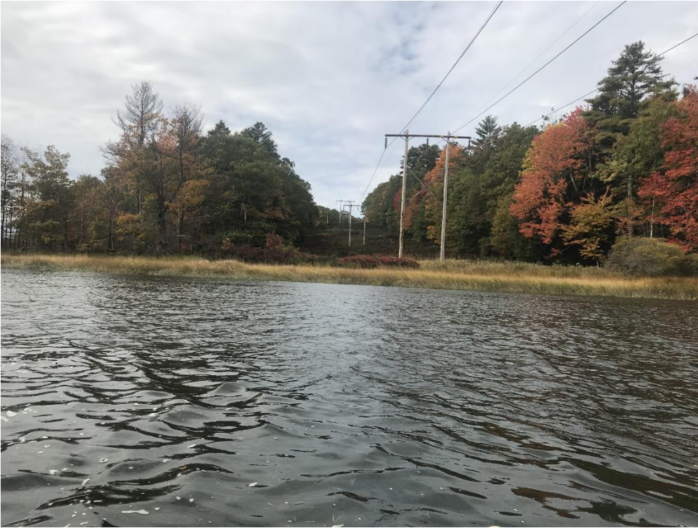
Photo 42: CMP powerline crossing
