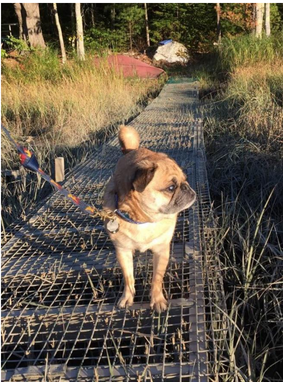
Photo 14: Steve Chef - walkway mowed/cut through saltmarsh (permanent structure laid into marsh grass as walkway & steps) - commenter, likely unpermitted
