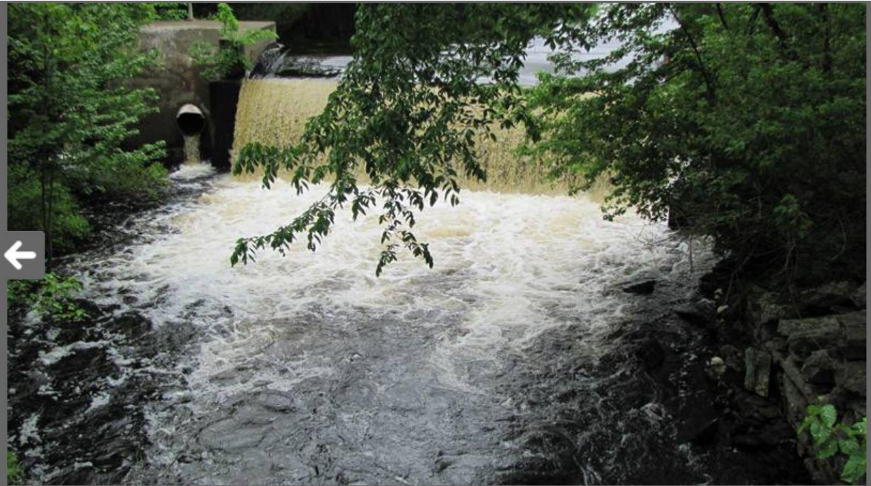
Dam at Coopers Mills (2012) Image 11 of 23
