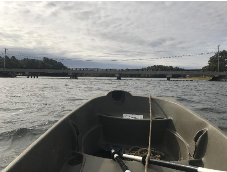
Photo 79: Sheepscot bridge (fixed bridge, ~6-8' vert clearance at high tide)
