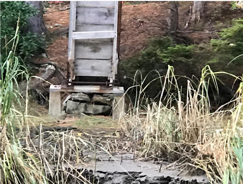
Photo 16: Lifted wooden dock/pier/floats with permanent concrete piers below HAT - (formerly Bill Mook) - Now Leah Sprague - commenter
