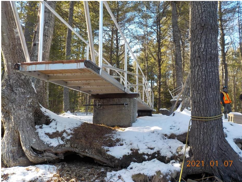
Photo 11: Granite block for gangway
