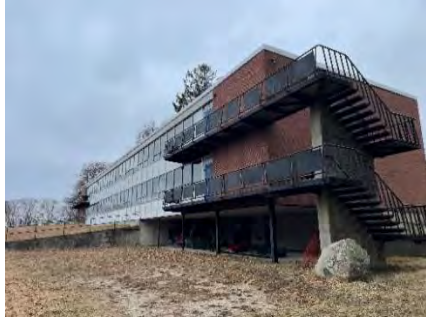
Canopy/overhang and exterior stair west side
