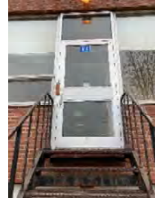
Exterior exit stair.
