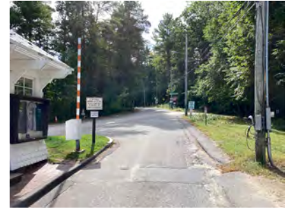
ISLAND ACCESS: GATEHOUSE
