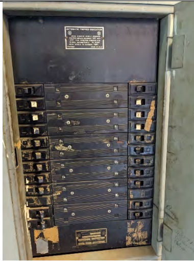
Deteriorated Panelboard
