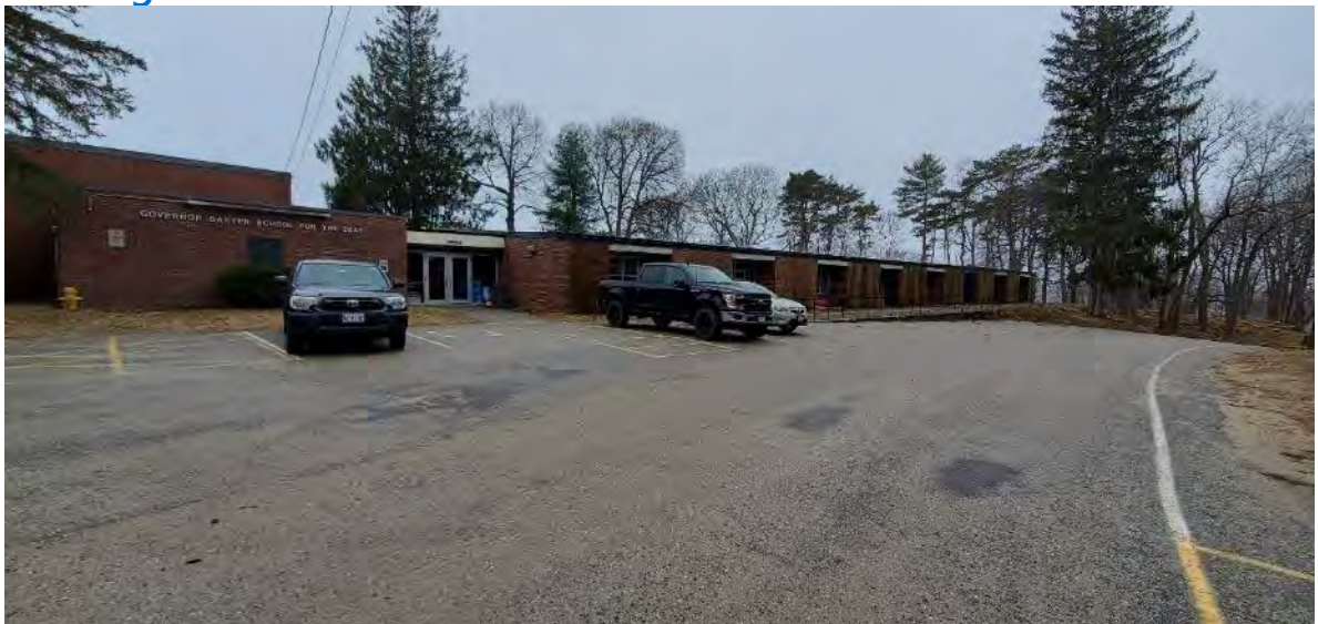
Photo 4: Building G: Carter parking lot
