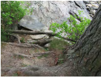
BLUFF EROSION AND LEDGE ARMOR
