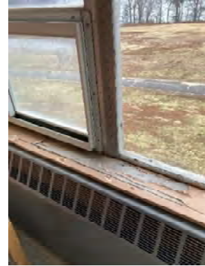
Water damage.
