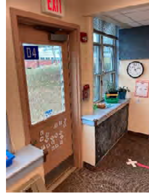
Grade-level exterior door.
