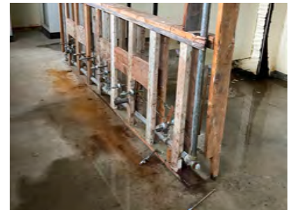
YOUNG: TOILET ROOM
