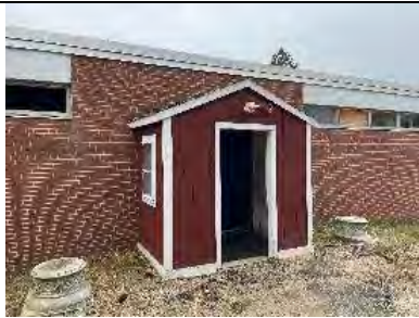
T-1-11 entry vestibule.
