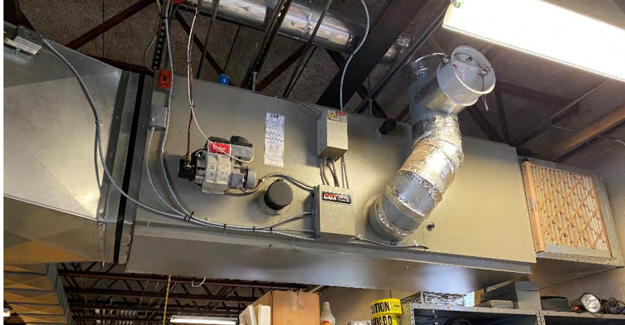
Figure 3 - Oil-fired Furnace
