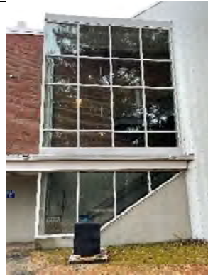
Curtain wall at egress.
