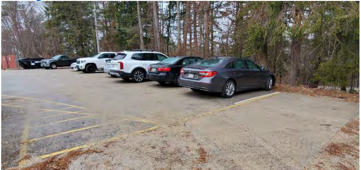
Photo 6: Building K: Sanders parking lot
