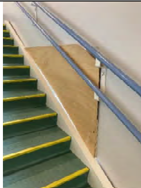
Main stair window protection.
