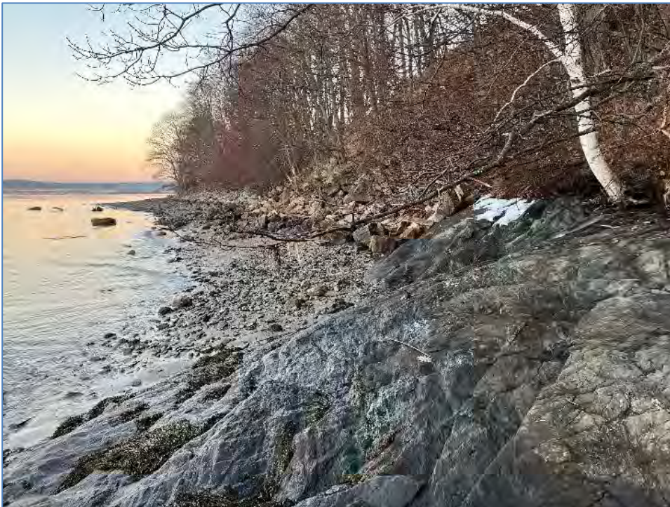
Fig. 15. Natural Ledge and Imported Riprap Protect the Coastal Embankment
