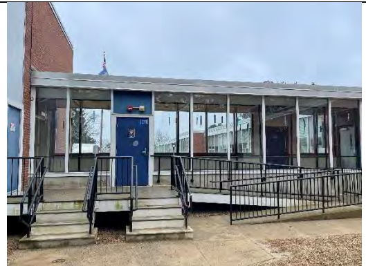
Exterior stairs and ramp.
