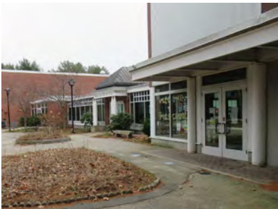
MAIN SCHOOL ENTRY
