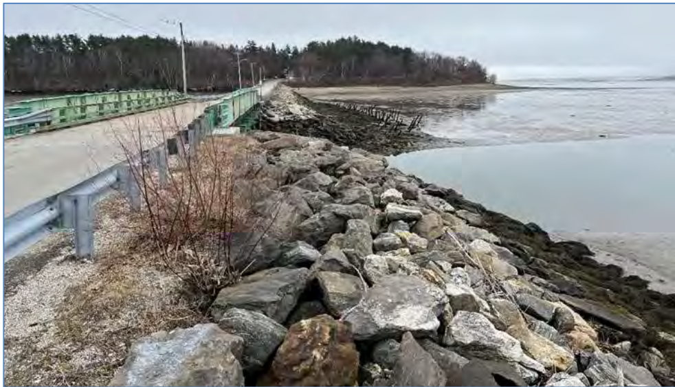
Fig. 10. Mackworth Island Bridge Looking East from Mainland
