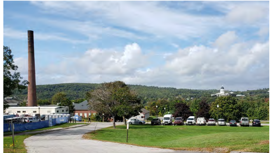
▲ East Campus with Capitol Building in Background
