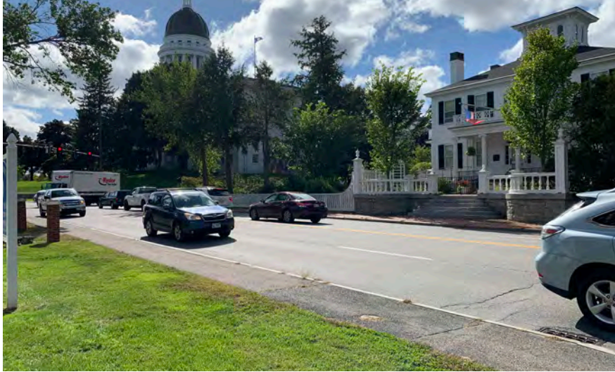
▲ Existing vehicular access, West Campus
