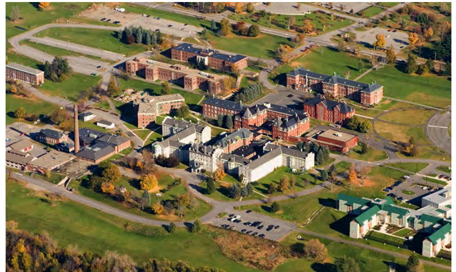
▲ East Campus Aerial
