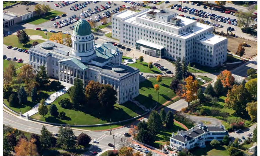
▲ West Campus Aerial
