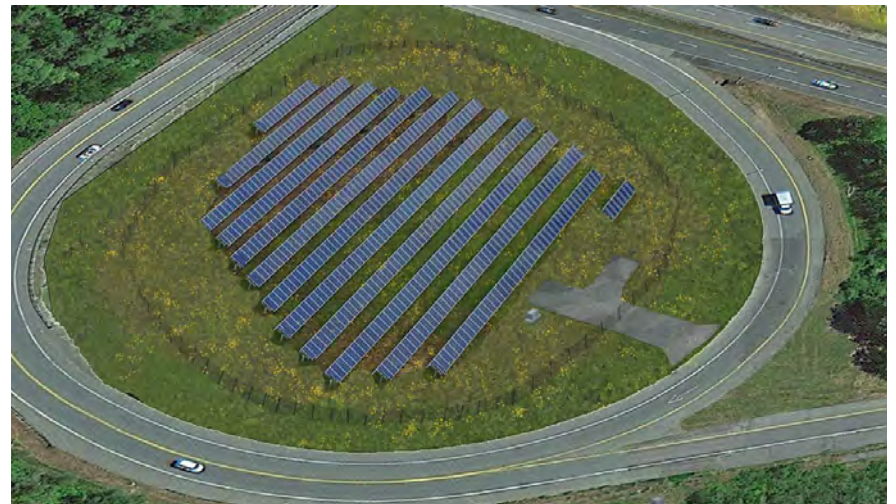
▲ Maine DOT solar installation along I-95.
