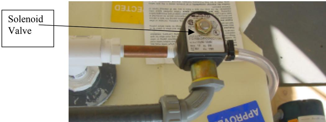
Figure 3: Normally closed solenoid valve
