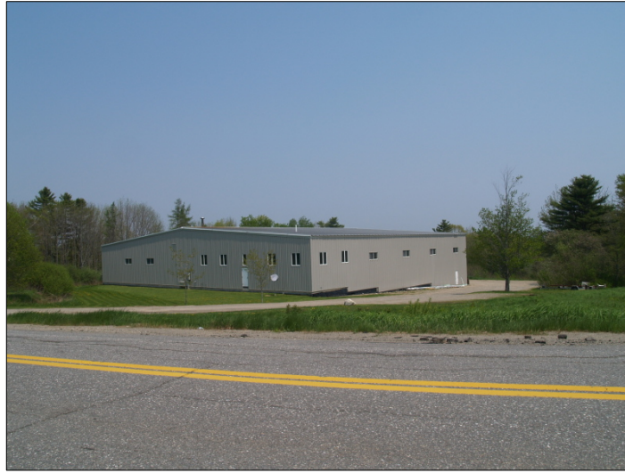
Building fully exposed to view.
