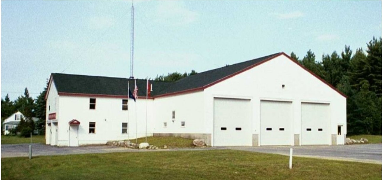
Spurr's Corner Fire Station
