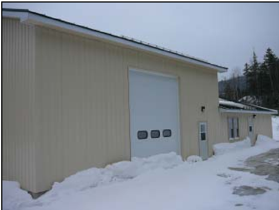
Operations and Maintenance Building (back view).
