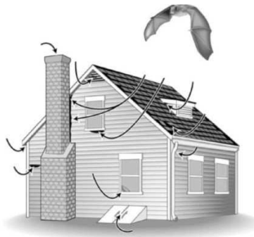
Common entry points on homes and buildings include corners, eaves and louvres.
