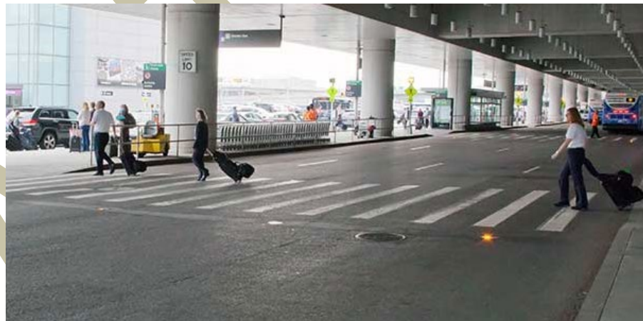
Figure 12 – In-Road Pedestrian Lights
