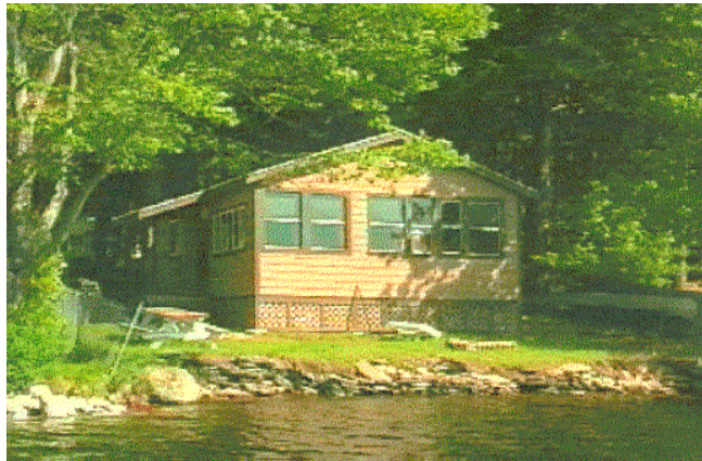
A typical lake front cabin with hardly any buffer. The owners are growing a lawn on the narrow space between the cabin and the lake.
