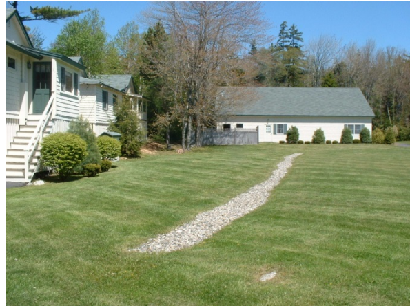
Figure 6.4 - Photo of Infiltration Trench
